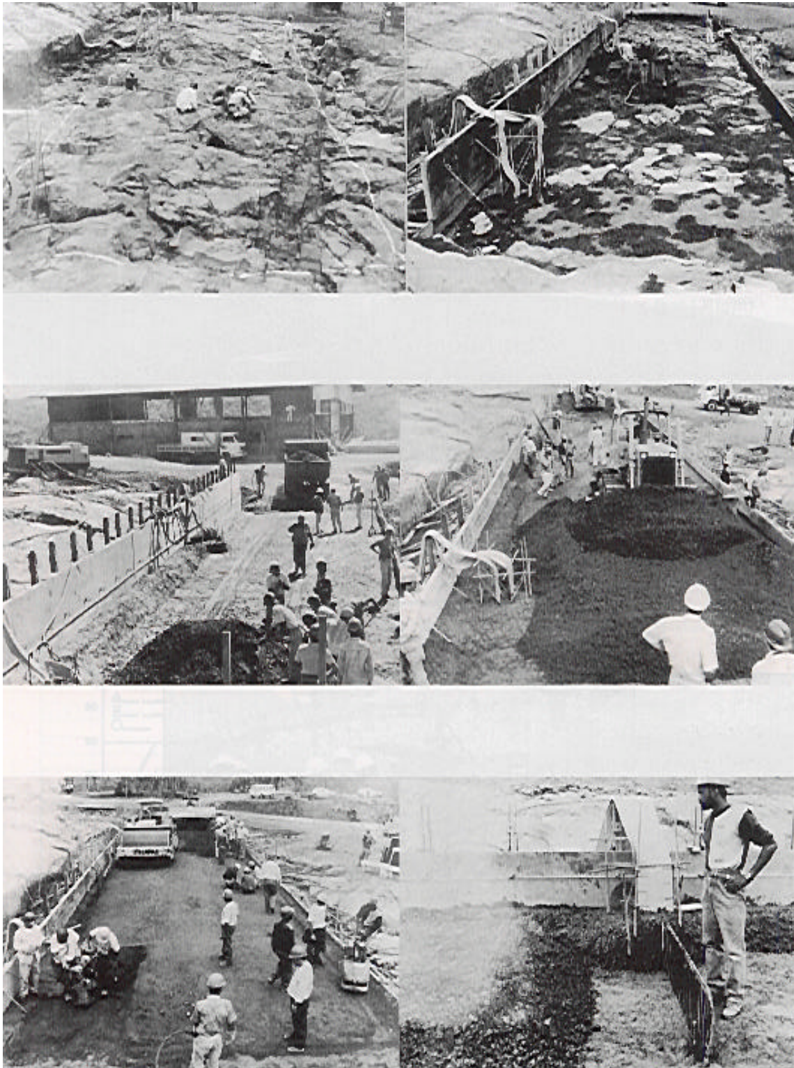
FIGURE 10- General View of the Test Fill during the execution- Foundation Preparation; Forms Preparation; Face Mix & Bedding Mix placement; Spreading RCC; RCC Compaction; Contraction Joint Form-Inducer.
