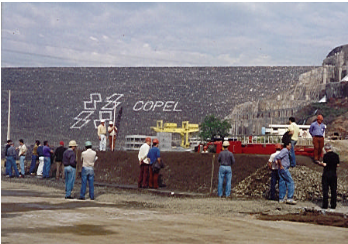
FIGURE 1- Tests during the construction of the first test fill- JUNE/1993.
