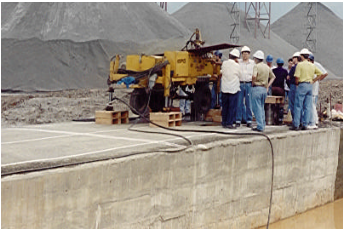
FIGURE 12- Drilling cores from the Test Fill on delimited regions
