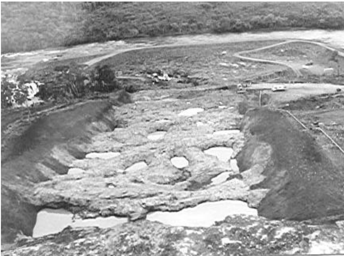
FIGURE 10 - View of the irregularities observed at the left abutment
