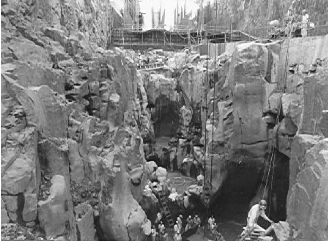
FIGURE 6- Cavities at the foundation rock right at the downstream Sluiceway
