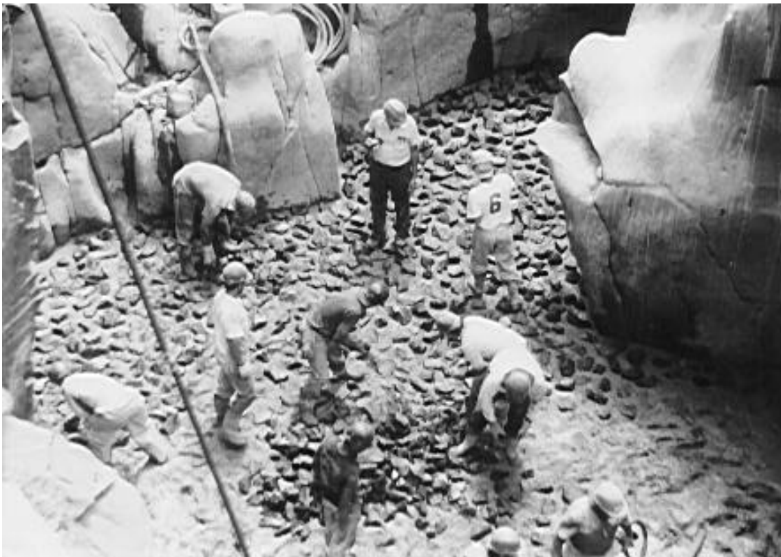
FIGURA 9- Condition observed during the filling of the cavities near the Sluiceway
