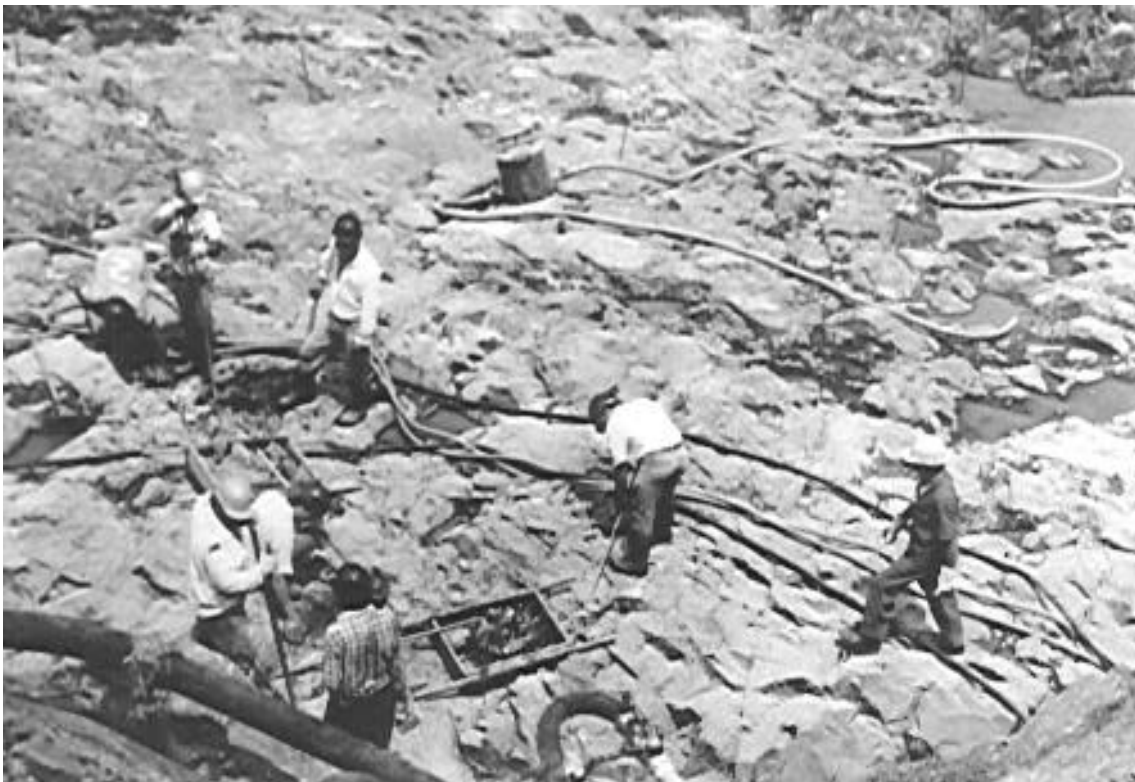
FIGURE 3- Very Irregular surface at river bed area
