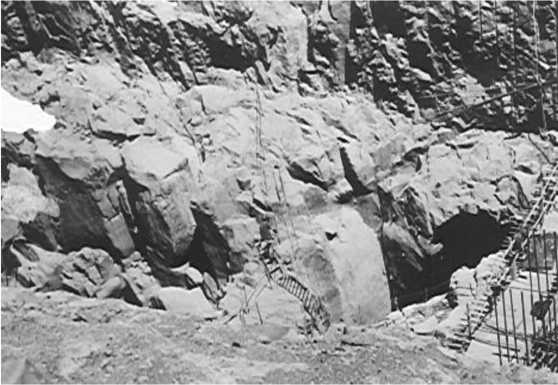
FIGURE 7- General view of cavities preparation downstream the Sluiceway
