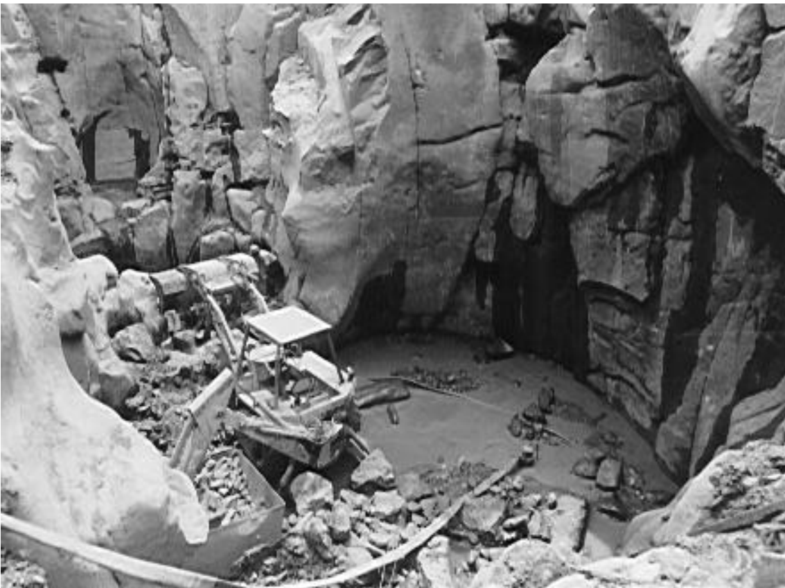
FIGURE 8- Equipment used for cavities' cleaning
