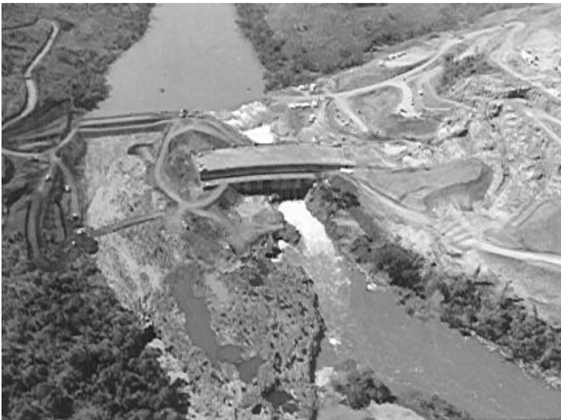
FIGURE 11- Aerial View of Dam construction by April/1995
