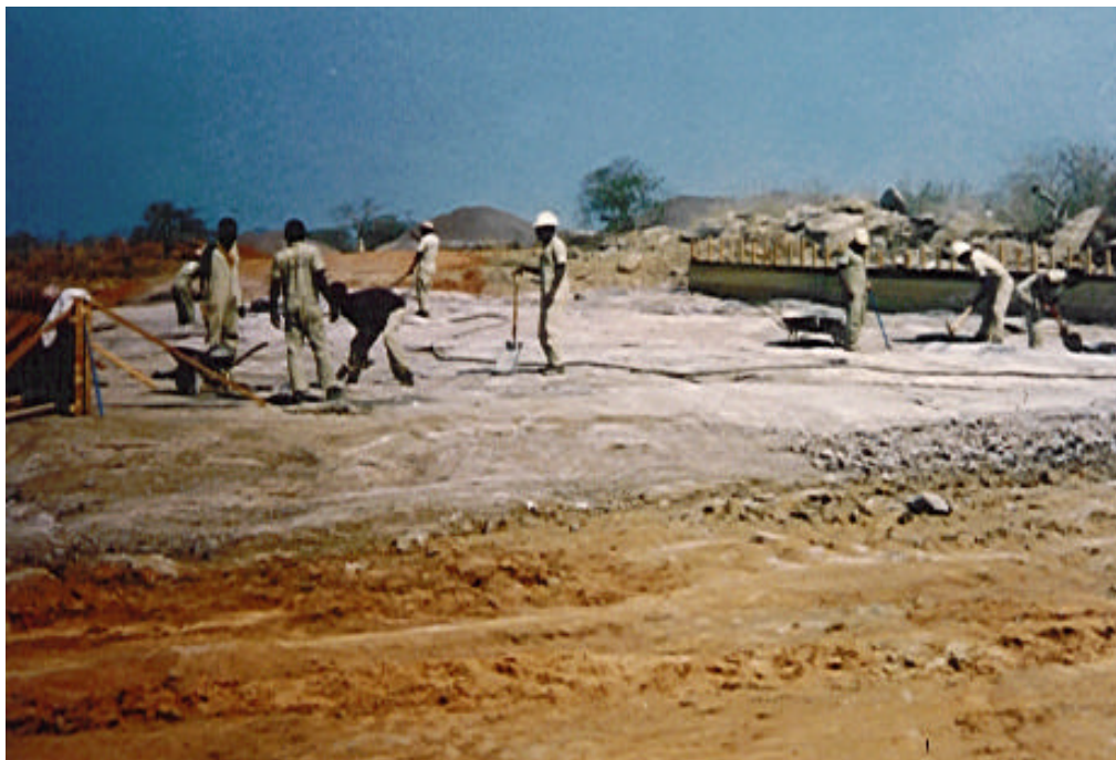
FIGURE 8- ROCK SURFACE PREPARATION FOR RCC-TEST FILL , AT CAPANDA JOB SITE
