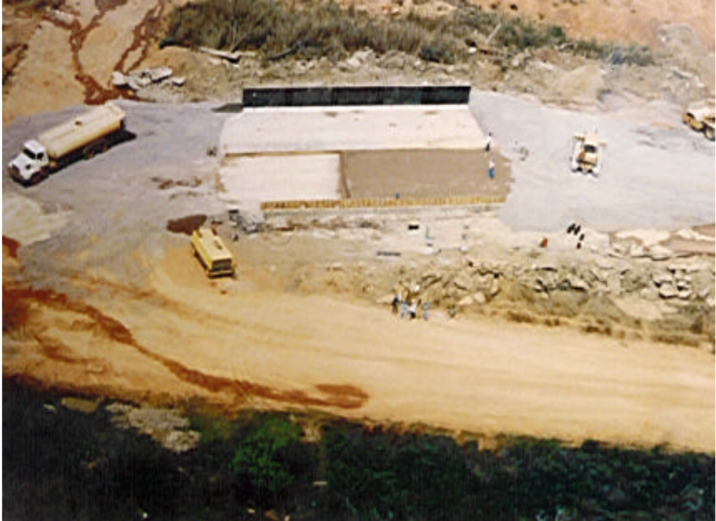
FIGURE 9- RCC PLACEMENT AT THE TEST-FILL, AT CAPANDA JOB SITE
