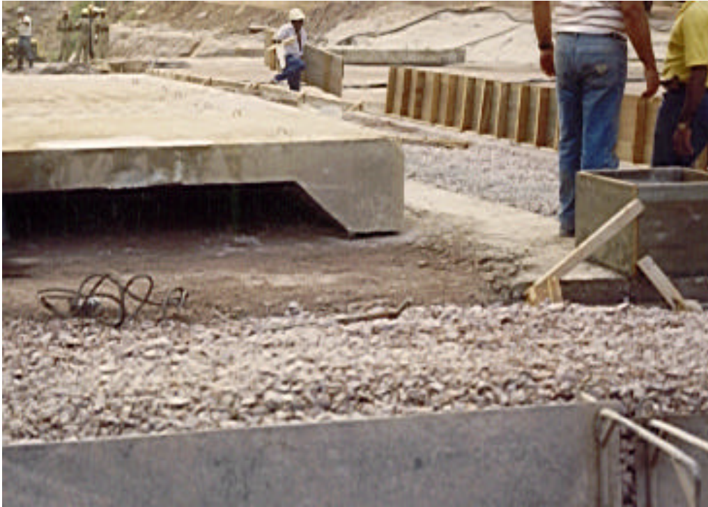
Figure 4 - Precasted concrete piece for the ceiling of the gallery
