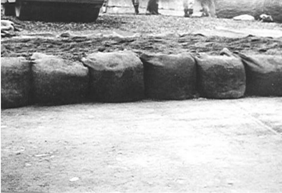
Figure 6 - Containers with granular material for casting the gallery
