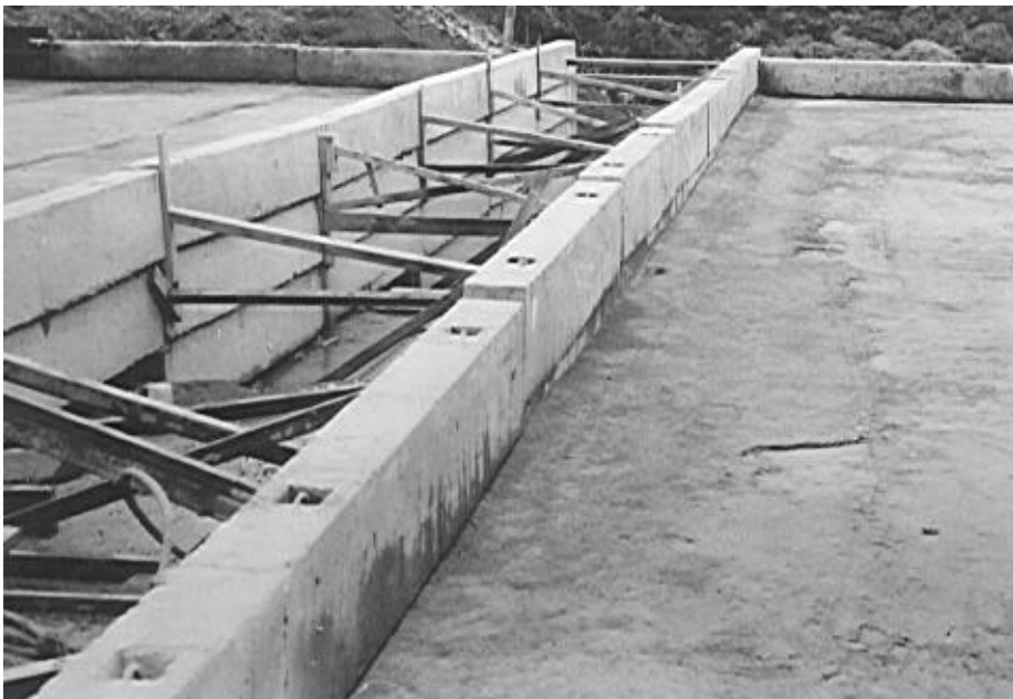
Figure 2 - Precasted concrete pieces for the shaping of the gallery
