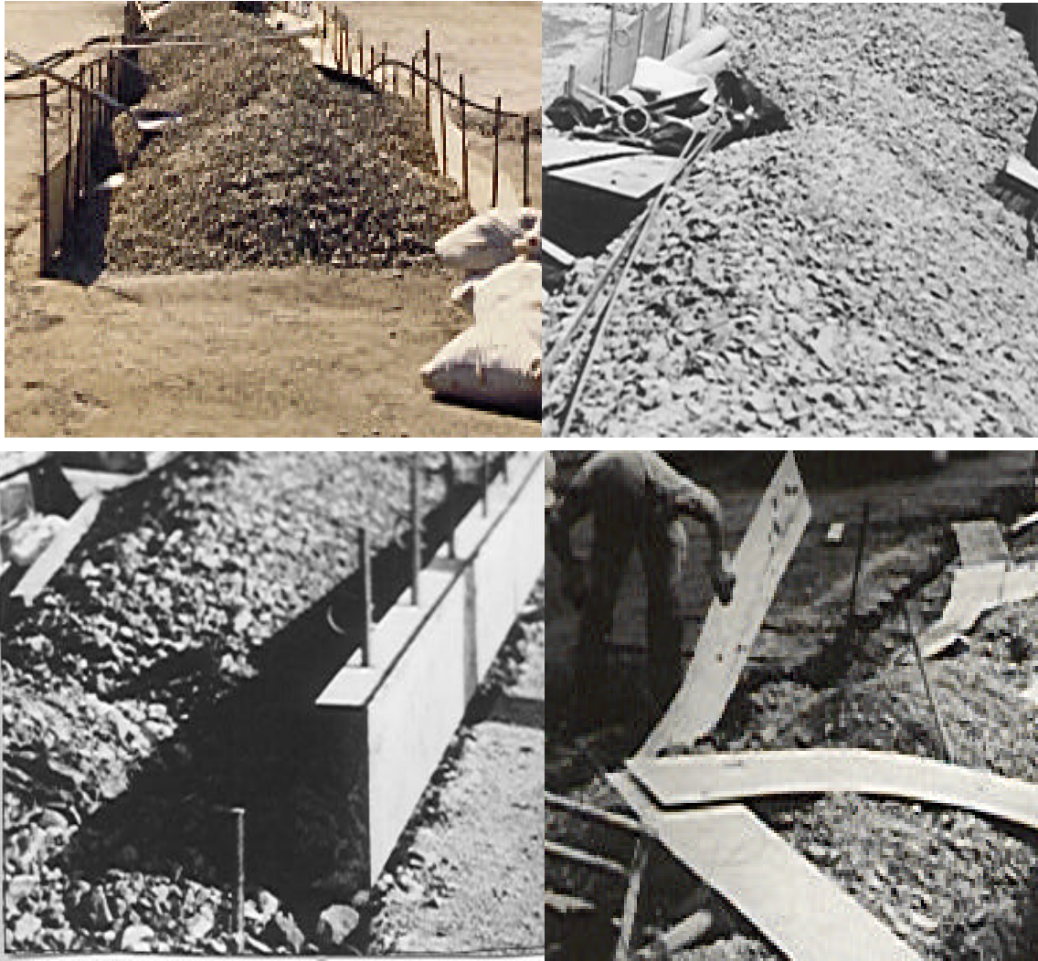
Figure 3 - Shaping of the gallery with granular material against wooden or metal forms
