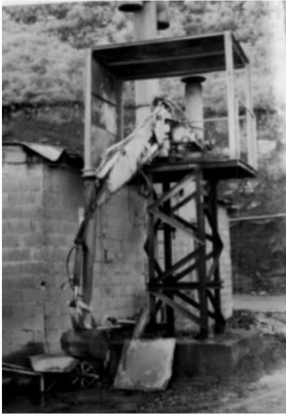
Figure 5.03- Sampler used at CVC and RCC Continuous Plant
