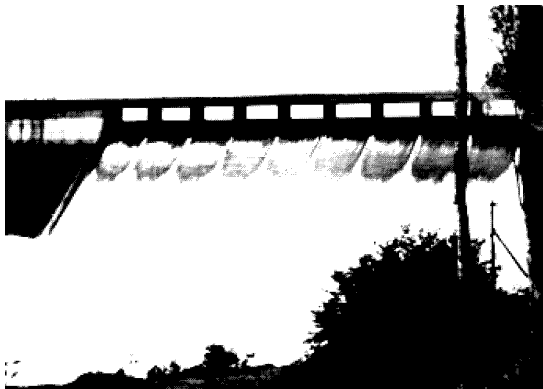
Figure 2- Urugua-i Dam (Argentina)
