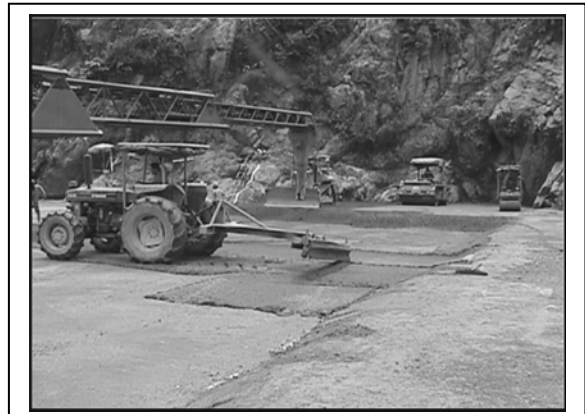
Figure 16- Spreading the bedding mortar
