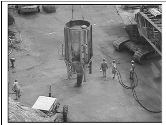
Figure 15- Bedding mortar delivery
