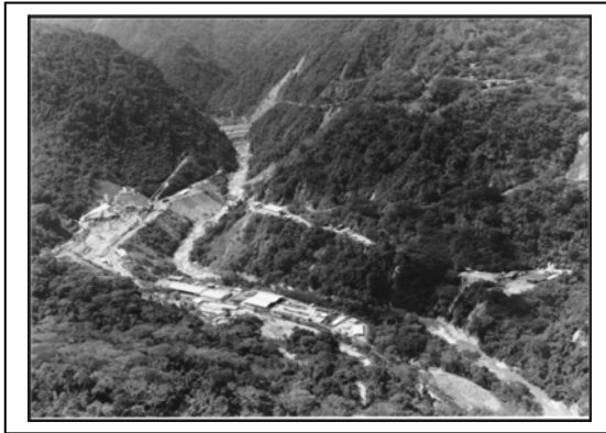
Figure 01- Overall view of the Project Site
