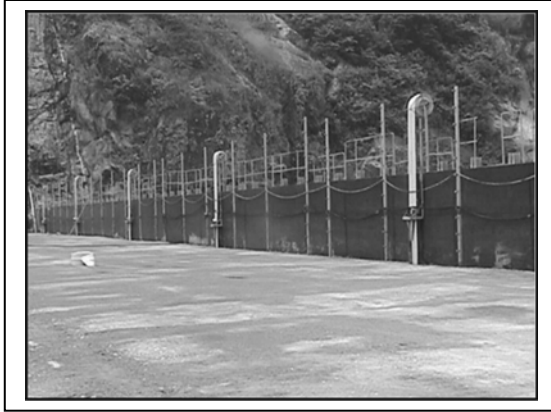
Figure 27- Upstream formwork and PVC membrane anchors
