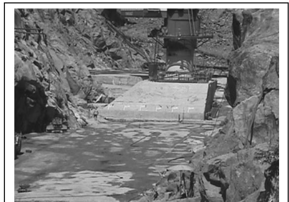
Figure 10- Assembling the Tower Belt
