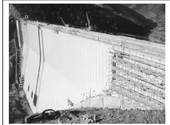
Figure 28- PVC membrane installation
