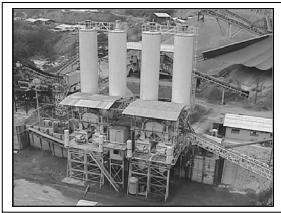
Figure 03- Overall view of RCC Plant
