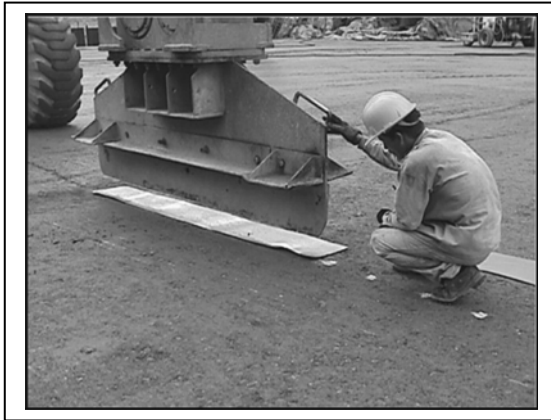
Figure 23- Metallic plate and Joint Inserter
