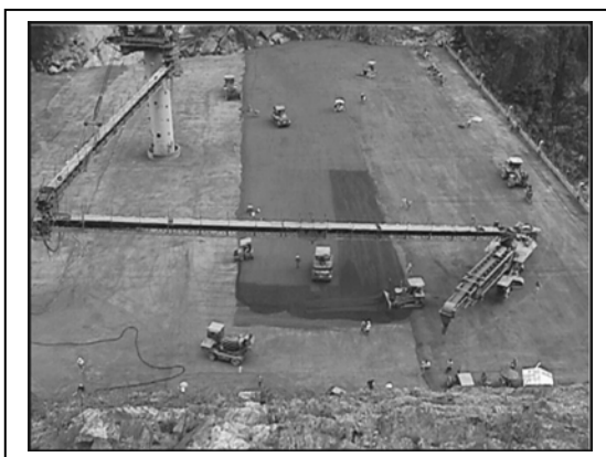
Figure 17- Overall view of RCC pouring
