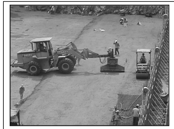
Figure 26- Overall view at upstream face
