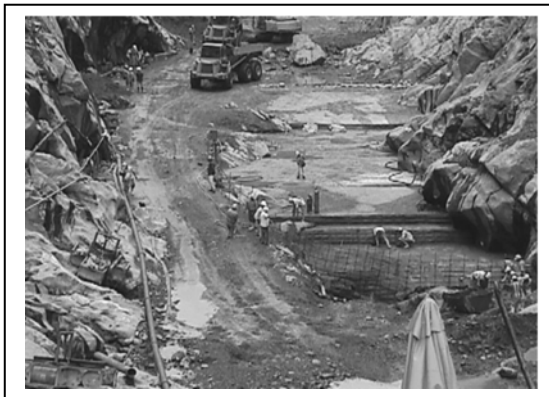
Figure 07- Dental concrete on river bed
