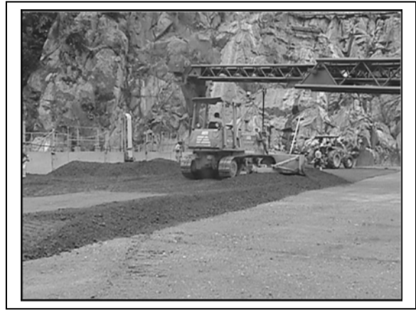
Figure 14 – RCC spreading and leveling
