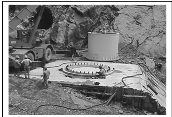
Figure 08- Tower Belt Crane base
