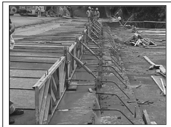
Figure 30- Downstream formwork system overall view
