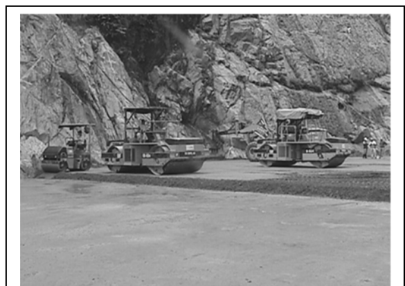
Figure 18- RCC compaction
