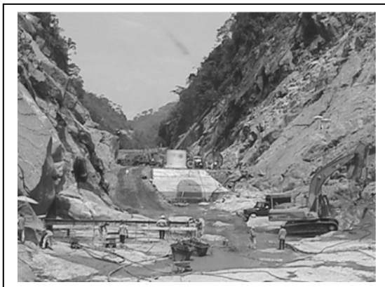
Figure 09- Overall view from foundation
