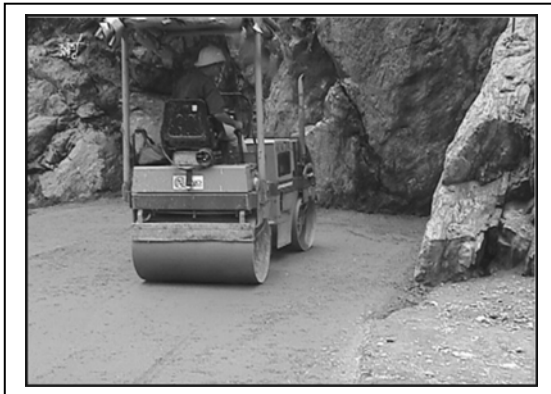
Figure 21- RCC compaction in confined zones
