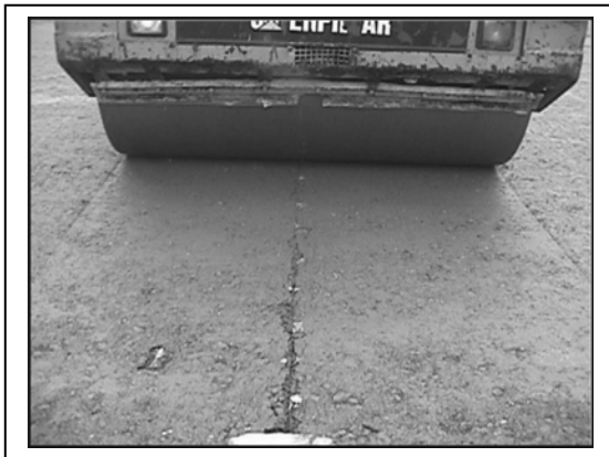
Figure 25- Finishing the contraction joint
