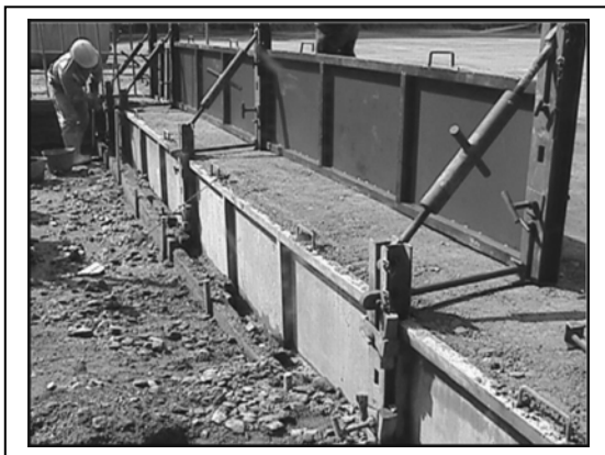
Figure 29- Downstream formwork system close view
