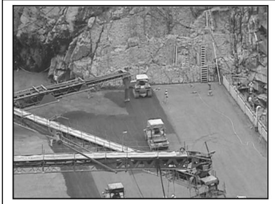
Figure 19- RCC spreading and compaction
