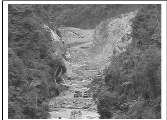
Figure 06- River bed excavation of the
