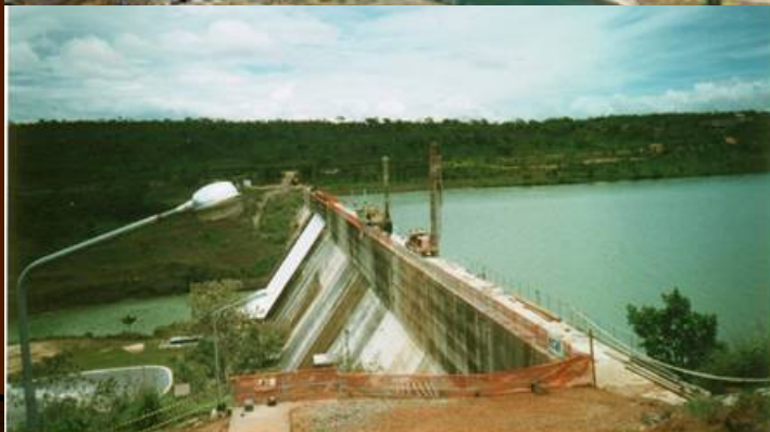
CHEMICAL EXPANSION OF CONCRETE IN DAMS & HYDRO-ELECTRIC PROJECTS
