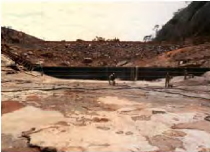
Figure 8.59 Foundation preparation at Capanda dam-Angola.
