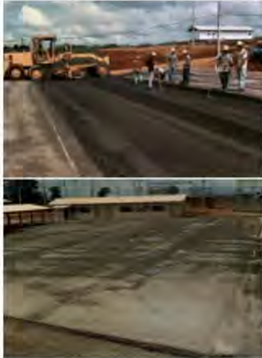
Figure 11.11 RCC used as stock pavement in Salto Caxias dam, Brazil.
