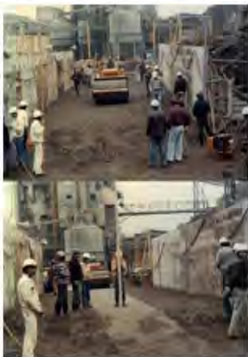
Figure 9.39 Test Fill Section at Itaipu (1977)- Topographic survey to check the number of roller passes and RCC top of layer settlement.
