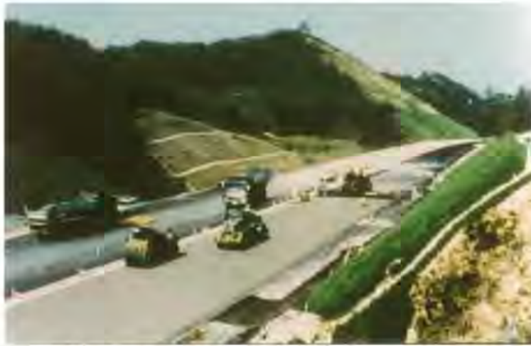
Figure 11.13 RCC used for road pavement in Japan. (Courtesy: Carlos Jofré - IECA)
