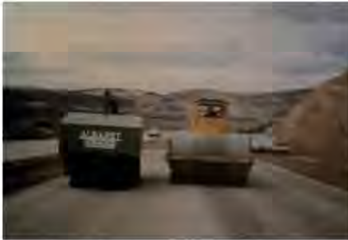
Figure 11.12 RCC used for road pavement in Spain. (Courtesy: Carlos Jofré- IECA)
