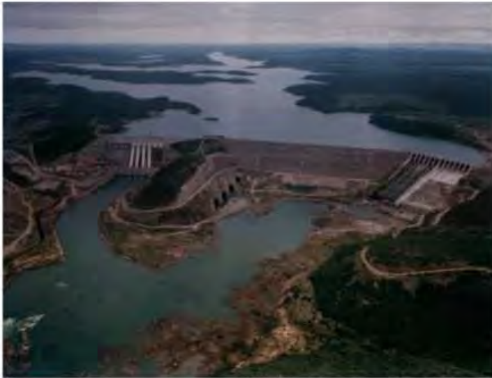
Figure 11.06 Overtopping protection at Xingó Dam by the end of construction, Brazil. (Courtesy: Alberto J. Cavalcanti-CHESF)
