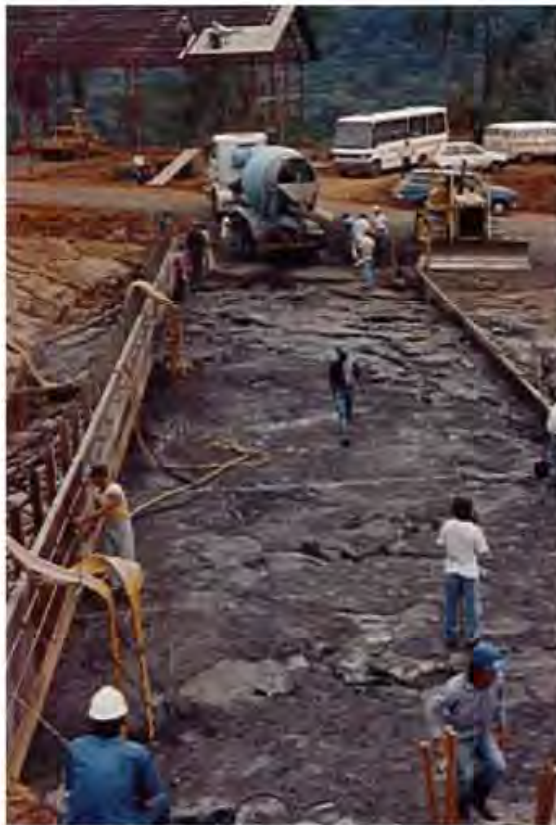
Figure 6.22 Preparation for a RCC test fill.
