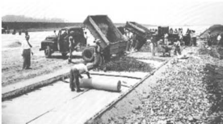
Figure 3.05 Paving works at Congonhas Airport (São Paulo, Brazil 1950). No-slump concrete [3-28].
