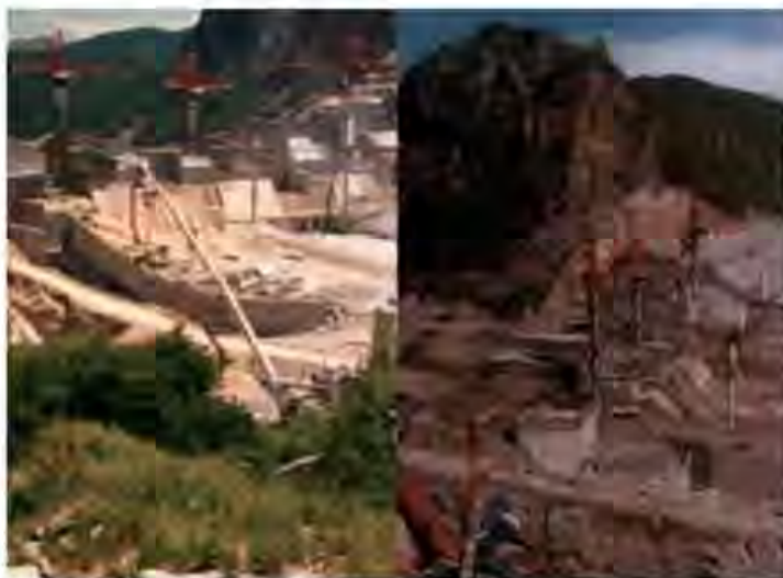
Figure 8.21 A modern system used for CVC placement at Huites (CVC mass concrete) dam-Mexico, at a monthly rate larger than 250,000m 3 .
