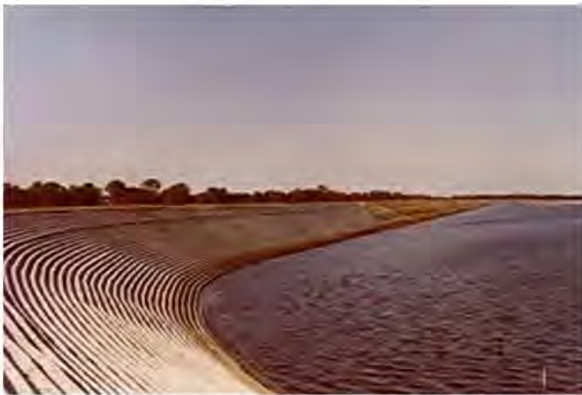
Figure 2.02 Soil (Gravel+Sand) Cement used as slope protection
