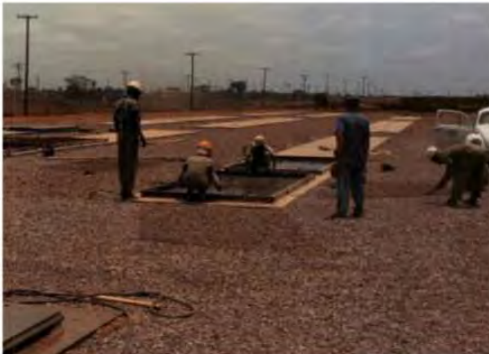
Figure 8.68 Element being cast with the PVC membrane as a (internal) face.
