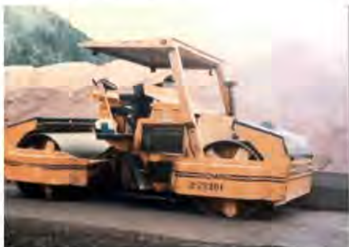
Figure 8.54 Wet RCC mixture giving wave aspect in front of the roller during compaction.
