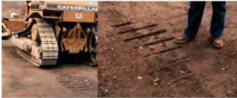
Figure 8.42 Damage caused on the RCC surface due to the dozer (heavier than necessary).
