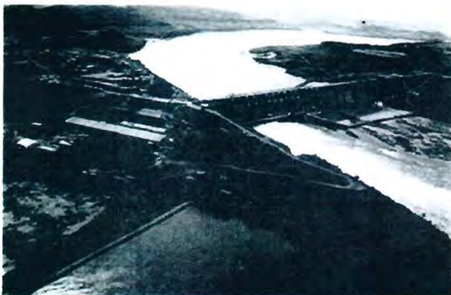
Salto Caxias , a 1240 MW Hydroelectric Power Plant, Iguaçu River – Brazil, with a 67 m high and 1 million m 3 RCC dam Basic and Detailed design by a Consortium led by INTERTECHNE – 1992/1998.
