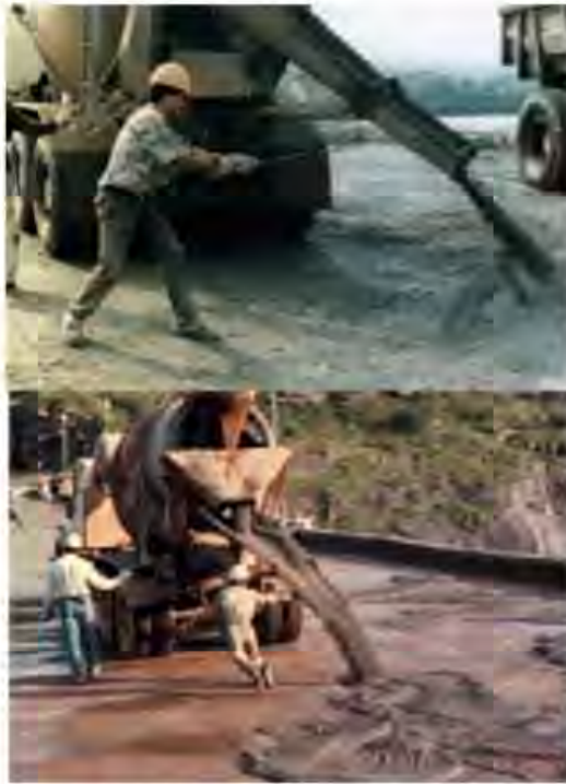
Figure 9.28 Bedding mix placed directly from the concrete truck-mixer.
