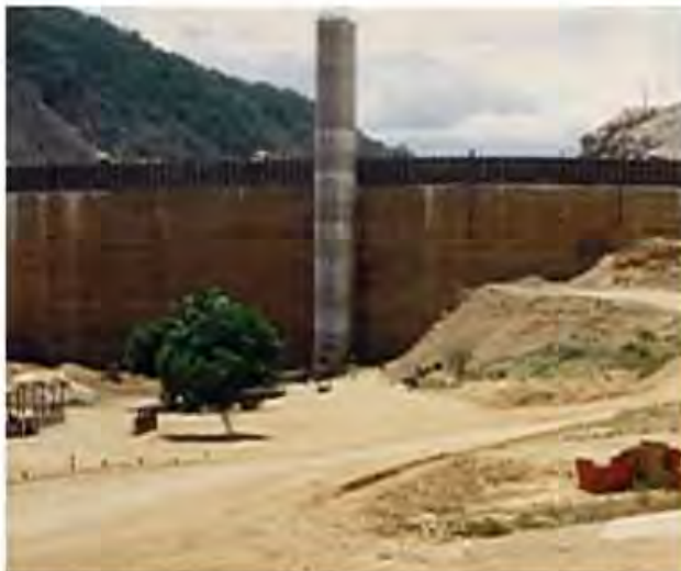
Figure 4.41 Diversion gallery and intake tower at Saco de Nova Olinda Dam.
