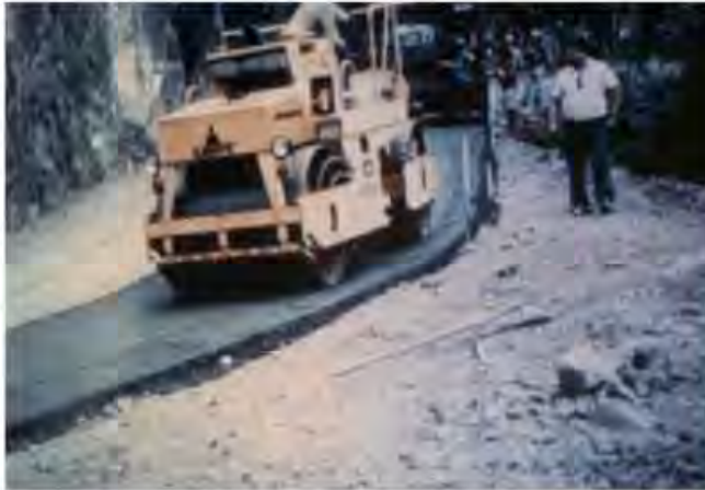
Figure 11.23 Road RCC pavement in Serra do Rio do Rastro, Brazil.
