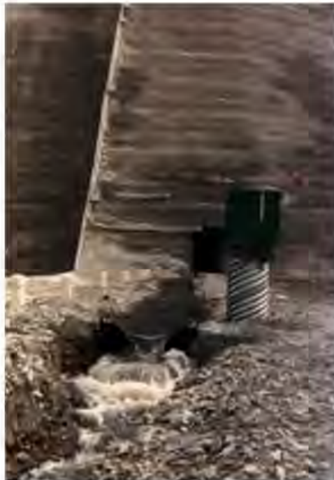
Figure 12.09 Leakage from the gallery at Galesville Dam (Courtesy: Selmo C. Kuperman).
