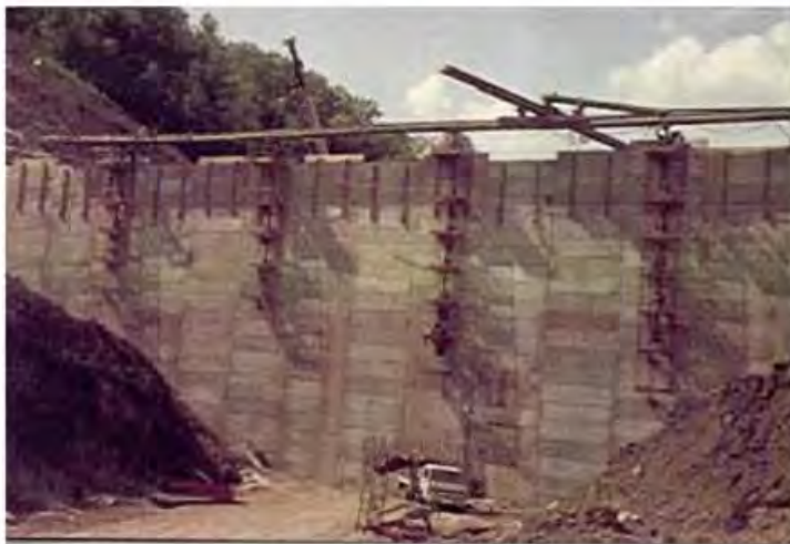
Figure 4.24 Precast concrete panel as form at Spring Hollow Dam (Courtesy: Rotec Industries).
