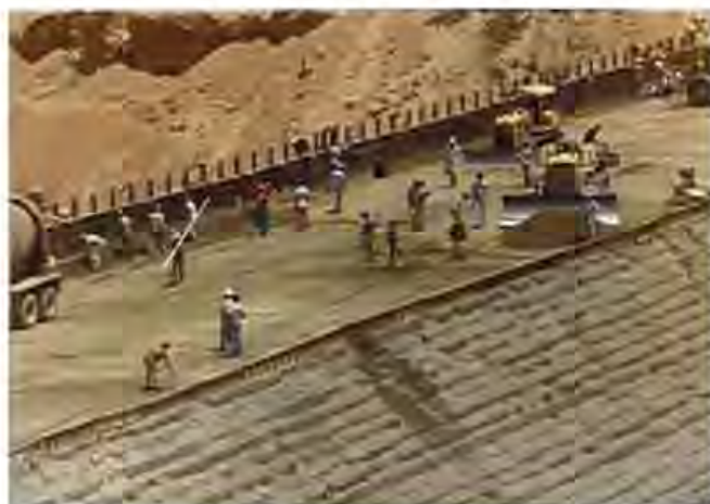
Figure 4.30 RCC cast against mould (cast-in-situ), for downstream face at Saco de Nova Olinda Dam.
