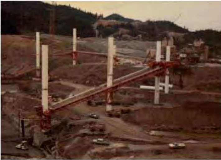
Figure 8.22 Belt conveyor used for RCC transportation and placement at Elk Creek dam (Courtesy: Rotec Industries).
