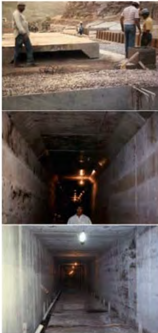
Figure 8.86 Pre-cast concrete piece for the ceiling of the gallery.
