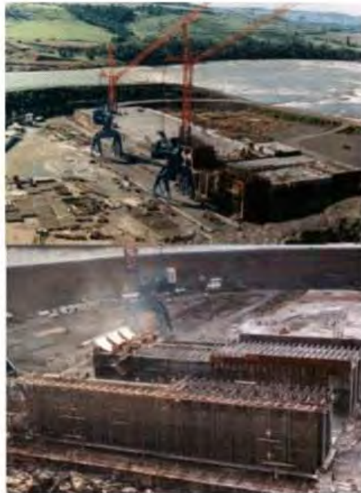
Figure 8.81 Diversion sluiceway built on CVC slipformed at Salto Caxias dam-Brazil.
