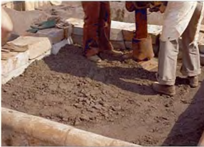
Figure 6.23 Trench at test fill during RCC compaction.
