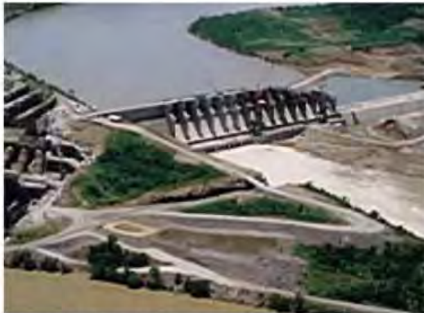
Figure 4.40 Salto Caxias Dam in Brazil- controlled spillway. Smoothed CVC concrete surface- Q_{\max} = 49,600 \text{ m}^3/\text{s} .
