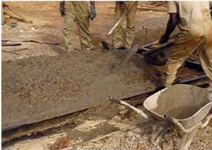
Figure 4.14 Concrete placement in the panel mould at Capanda Dam.
