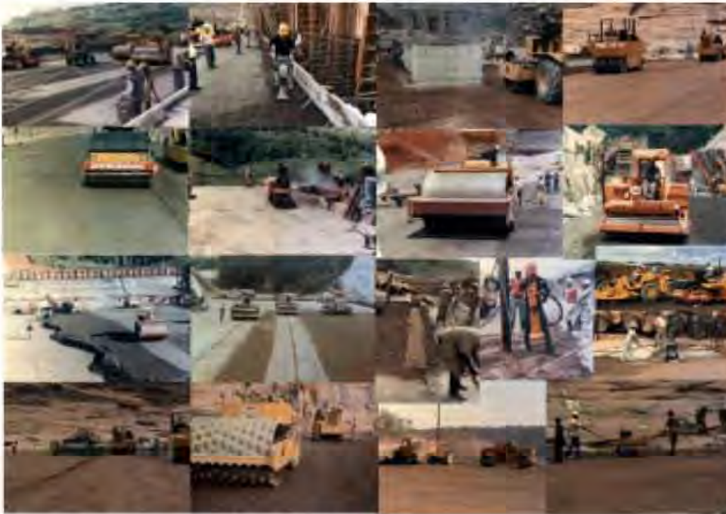
Figure 8.48 Equipment used for RCC compaction.
