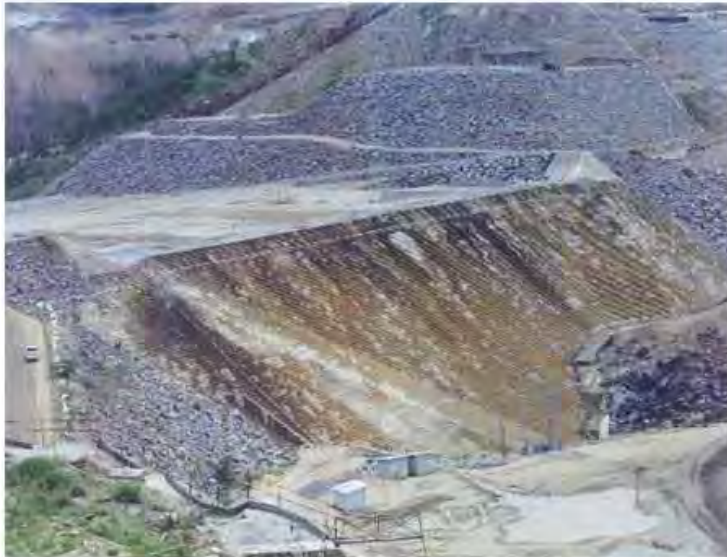
Figure 11.04 Overtopping protection at Xingó Dam during construction, Brazil. (Courtesy: Alberto J. Cavalcanti-CHESF)
