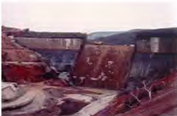
Figure 4.37 Caraibas Dam in Brazil- uncontrolled stepped spillway.
