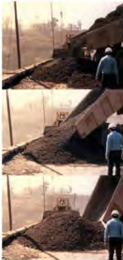
Figure 8.34 RCC dumped onto the uncompact material.
