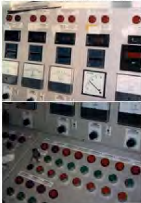
Figure 9.11 Control panel at RCC batching plant.
