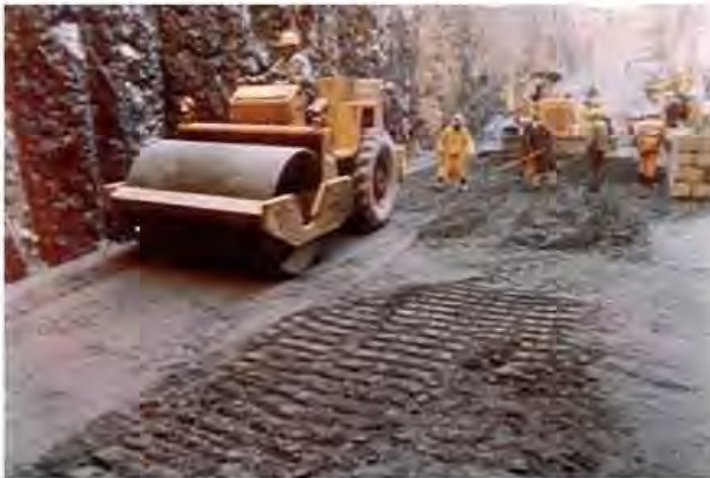
Figure 11.01 Backfill at downstream access ramp of Diversion Structure at Itaipu Dam.
