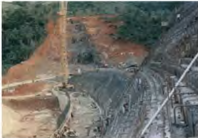
Figure 8.73 RCC poured directly against the form at a stepped downstream slope - Jordão dam-Brazil.
