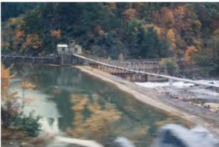
Figure 11.07 RCC used to increase safety during overtopping at Ocoee no. 2 Dam , a 9.1-m high rockfill.
