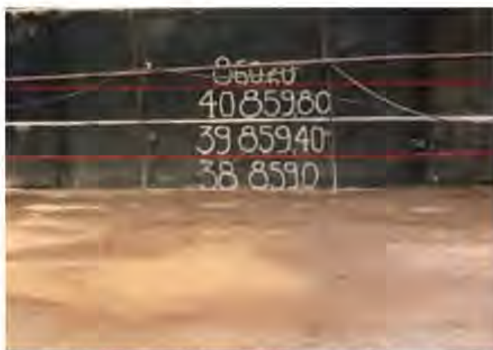
Figure 9.27 Horizontal reference strip painted at the upstream precast panel at Capanda Dam.
