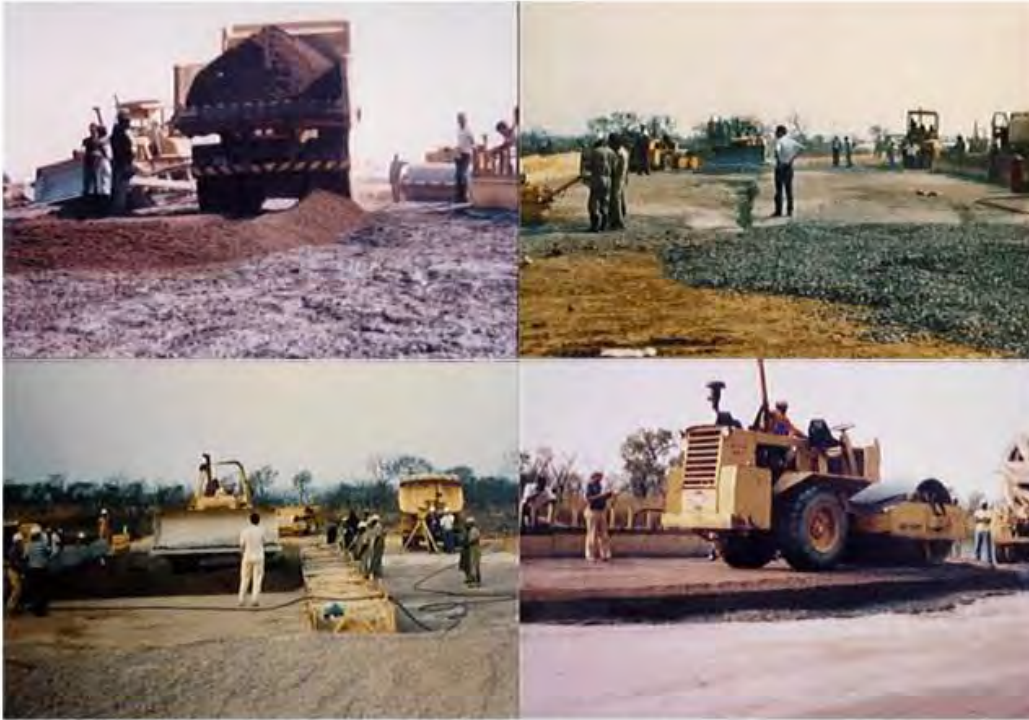
Figure 7.23 RCC placement at the test-fill at Capanda job site.
