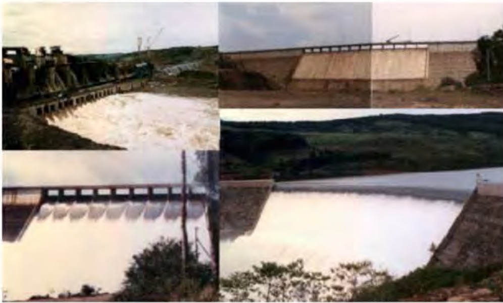
Figure 8.77 CVC smoothed spillway face at Urugua-i dam-Argentina, Jordão and Salto Caxias Dams - Brazil.
