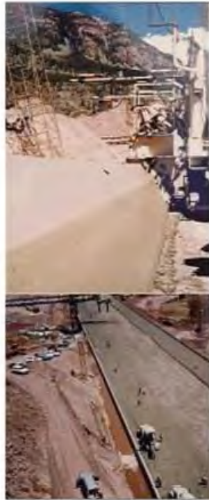
Figure 4.23 Upstream face being casted at Upper Stillwater Dam.
