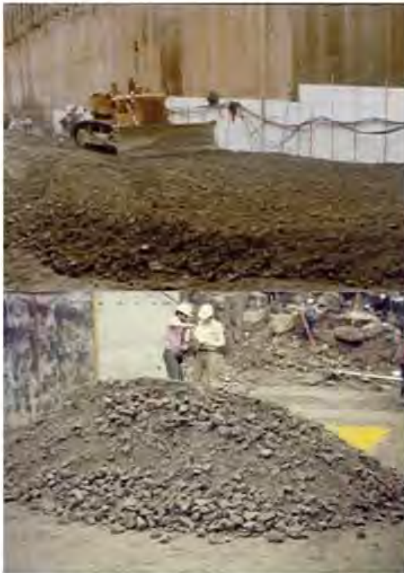
Figure 5.19 Segregation in RCC proportioned with the same content of 76mm aggregate as CVC.
