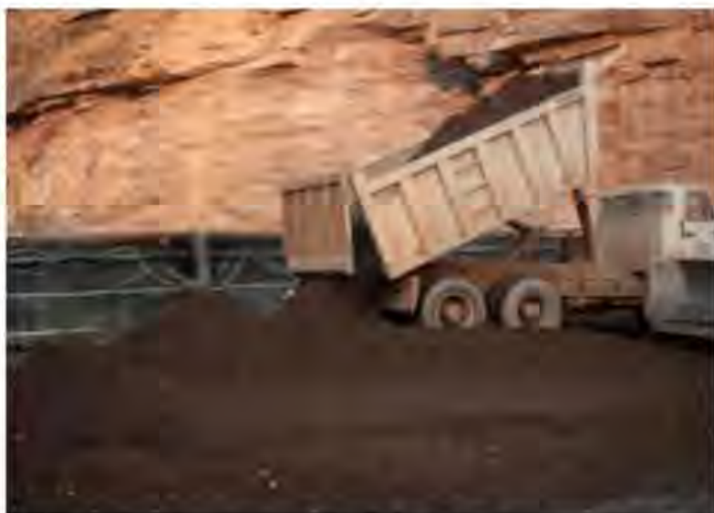
Figure 8.44 Material being dumped on top of the new lift being placed, allowing rework of slightly segregated dumped material.
