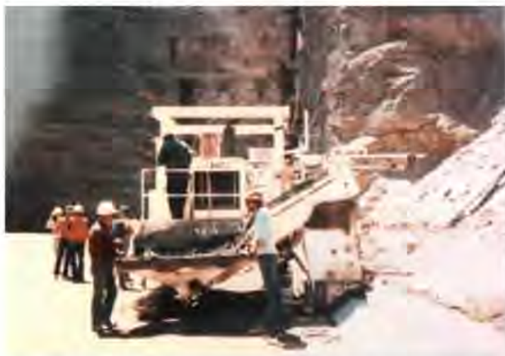
Figure 8.71 Dam face being cast by a powered curbing machine at Upper Stillwater dam-USA.
