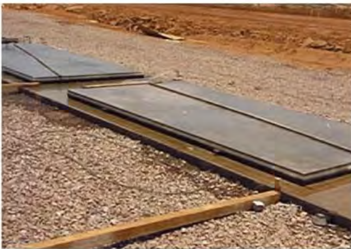
Figure 4.15 Precast concrete panel curing at Capanda Dam.
