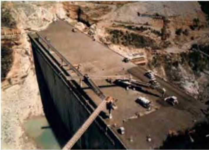
Figure 8.27 Belt conveyor used for RCC transportation and placement at Pangué dam (Courtesy: Rotec Industries).
