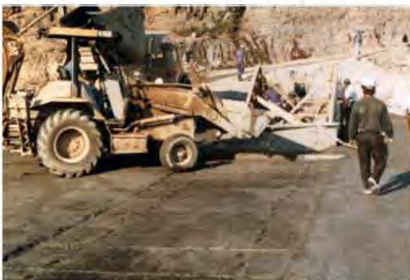
Figure 8.05 Gallery at a high level in a restrict area to RCC placement.
