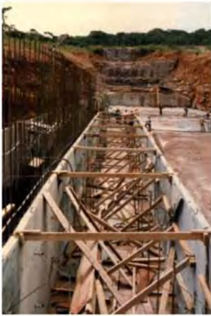
Figure 8.83 Pre-cast concrete pieces for the shaping of the gallery.
