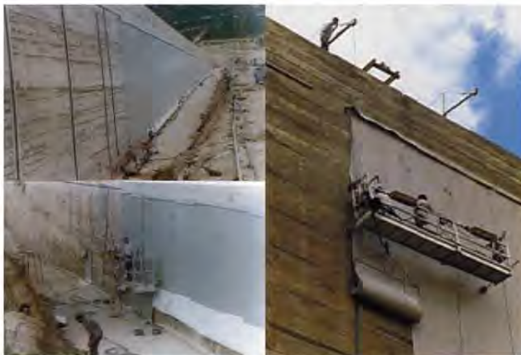
Figure 4.27 PVC membrane applied after the construction of Concepción RCC Dam (Courtesy: CARPI Systems).
