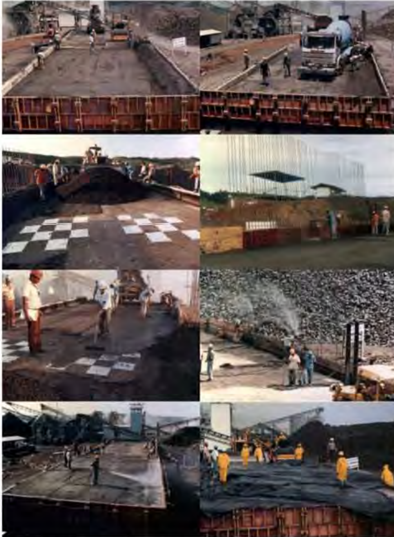
Figure 9.42 General View of the Test Fill during execution- Foundation Preparation; Forms Preparation; Face Mix & Bedding Mix placement; Spreading RCC; RCC Compaction; Contraction Joint Form-Inducer- Salto Caxias Site- Brazil (1996).
