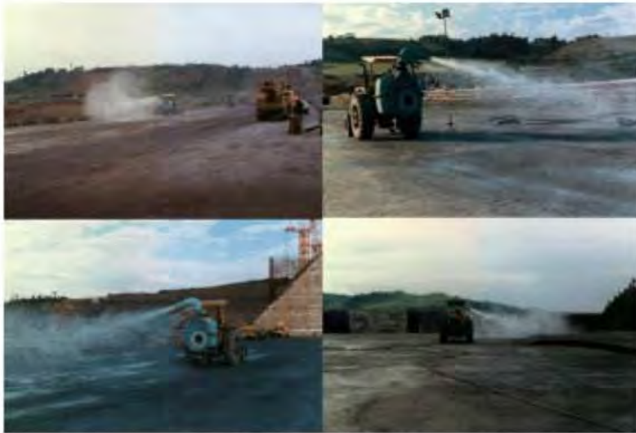
Figure 8.55 Fog spray during RCC placement and curing at Salto Caxias dam.
