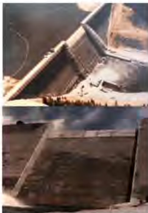
Figure 12.08 Seepage at downstream face at Galesville Dam (Courtesy: Selmo C. Kuperman).
