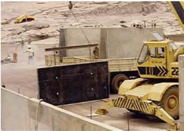
Figure 4.16 Handling and tilting up the precast panel at Capanda Dam.
