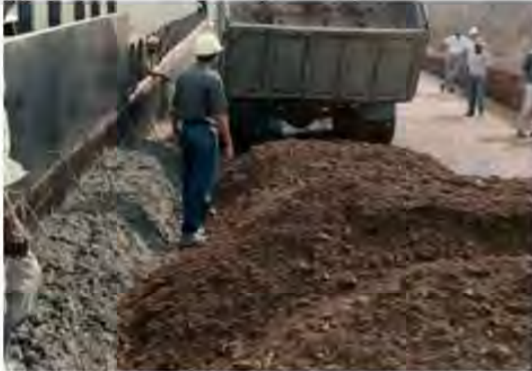
Figure 8.66 CVC being placed against form on the upstream slope, just ahead of the RCC placement.
