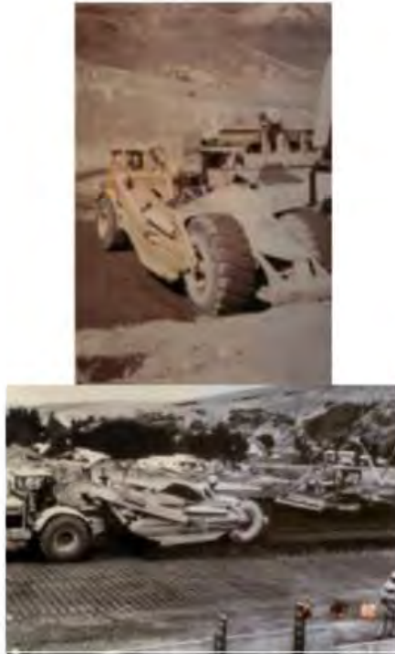
Figure 8.37 Scraper used for placing RCC, at Willow Creek dam-USA.
