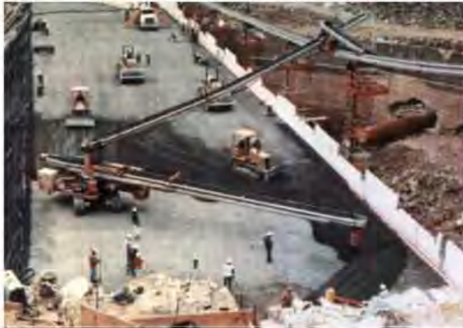
Figure 8.72 RCC poured directly, without form, on downstream slope.
