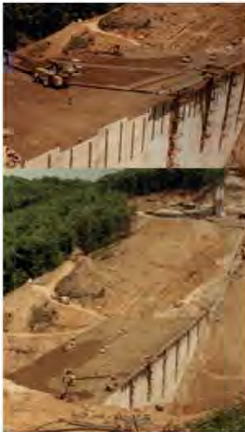
Figure 8.25 Belt conveyor used for RCC transportation and placement at Spring Hollow dam (Courtesy: Rotec Industries).
