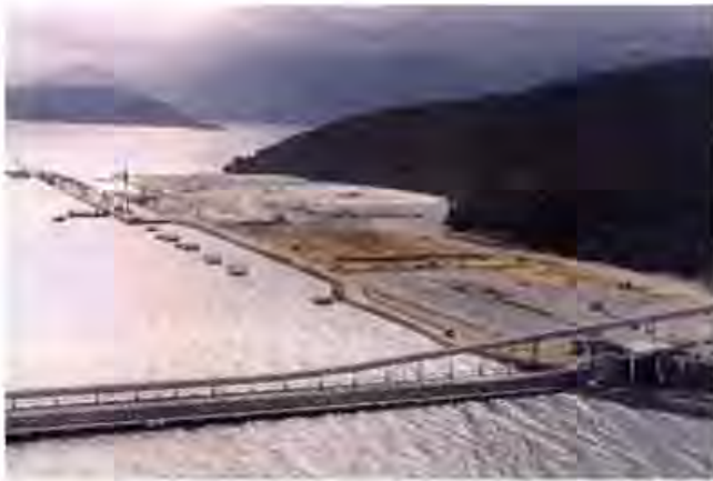
Figure 11.15 Aerial view of a bulk-terminal for cereals and minerals over a hydraulic earth-fill ( 2,700,000\text{m}^3 ) at Sepetiba bay, Rio de Janeiro, Brazil. (Courtesy: Carlos Yukio Suzuki-Planservi Engenharia Ltda.)
