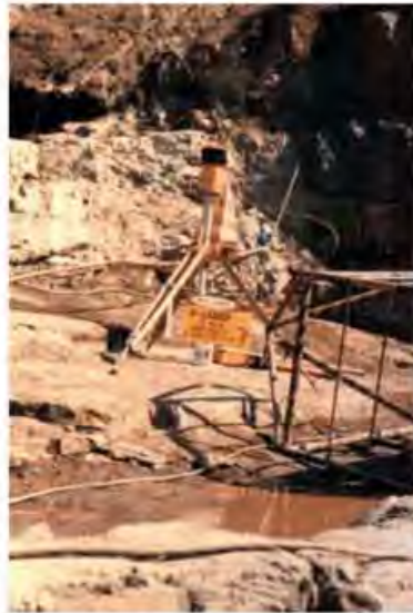
Figure 9.37 Laser ray for grade control at Urugua-i dam-Argentina.
