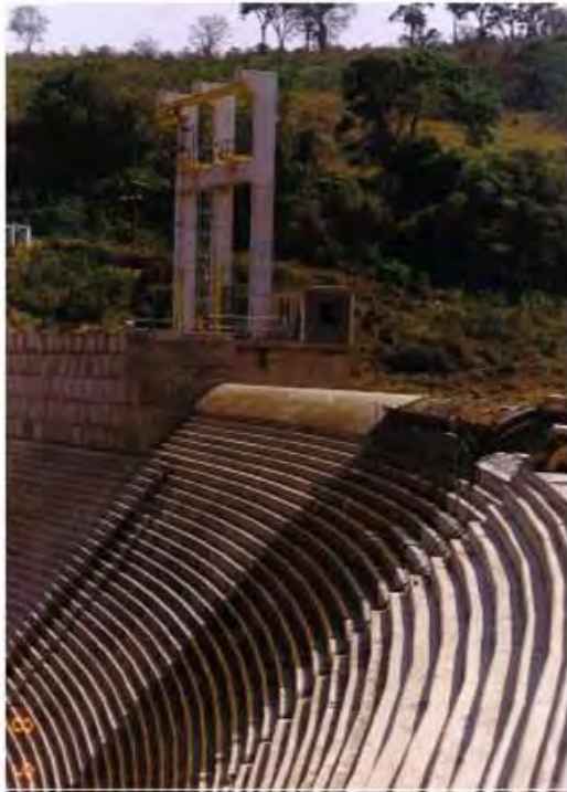
Figure 4.38 Rio do Peixe Dam in Brazil- uncontrolled stepped spillway.
