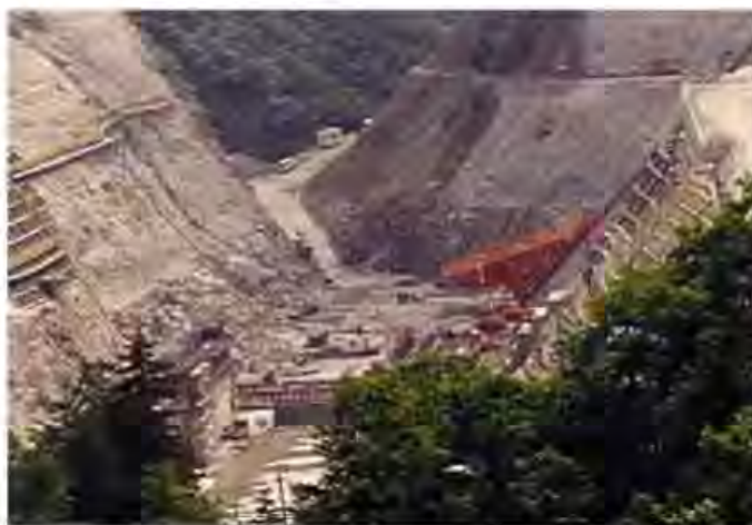
Figure 3.08 Sakaigawa RCD Dam, during construction, with contraction joints.
