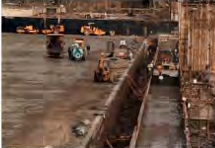
Figure 8.04 Gallery at a low level in a large area, ready to receive RCC.
