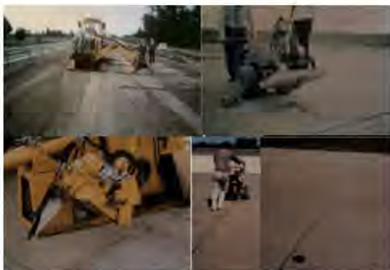
Figure 11.22 Joint cutting machines used for RCC pavement in Spain. (Courtesy: Carlos Jofré-IECA)
