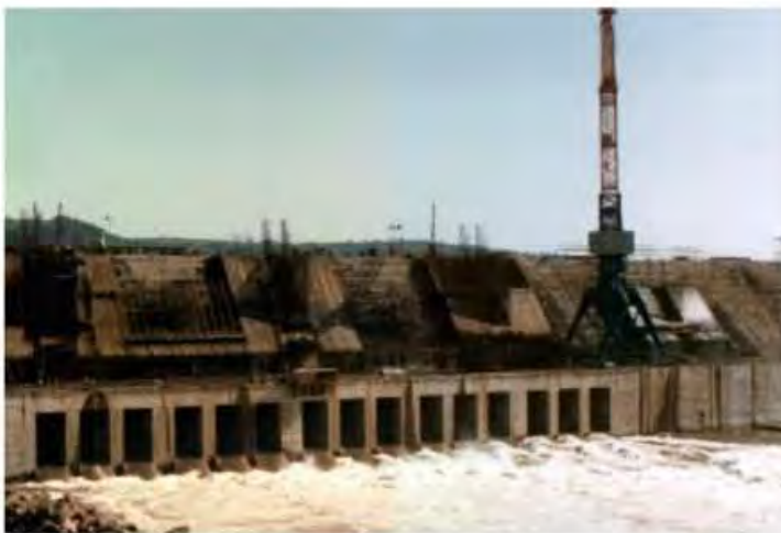
Figure 8.78 CVC smoothed spillway slab being cast over RCC dam body (and sluiceways) at Salto Caxias dam-Brazil.
