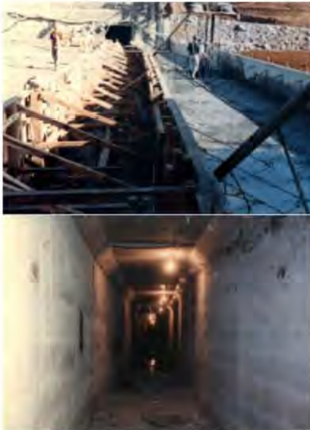
Figure 8.82 Gallery cast with RCC against conventional forms.
