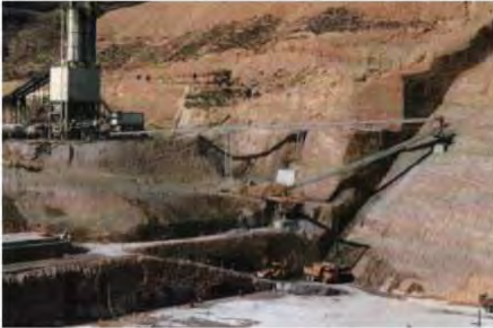
Figure 8.31 Belt conveyor used with a hauling vehicle for RCC transportation and placement at Val dam-Spain (Courtesy: Rotec Industries).
