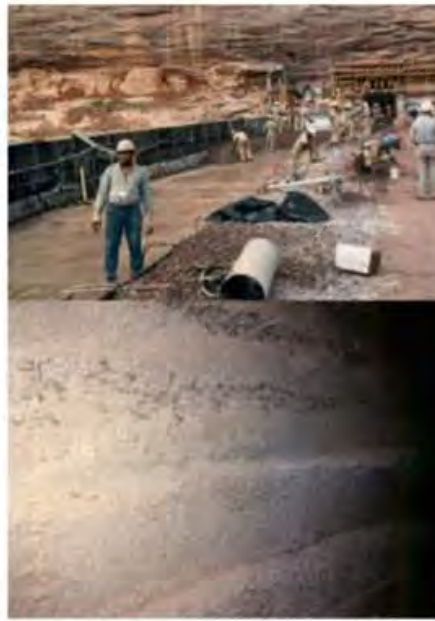
Figure 8.84 Shaping of the gallery with granular material against wooden or metal forms.
