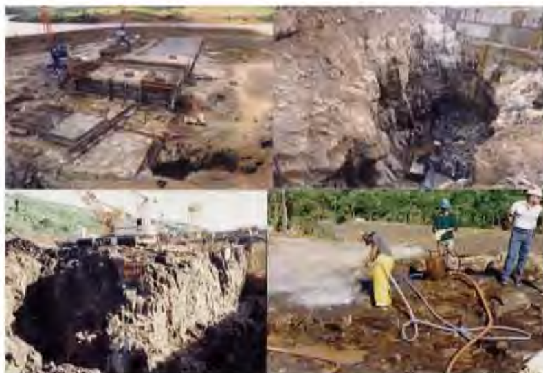
Figure 4.03 Some typical irregularities in basalt rock foundation - Jordão and Salto Caxias Dams.
