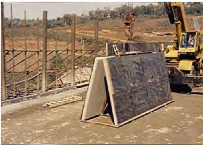
Figure 4.19 Precast concrete panel and the PVC membrane, bonded after the panel casting at Urugua-i Dam.
