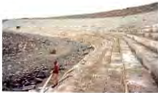
Figure 11.09 Wave protection at Porto Primavera Dam during construction, Brazil. (Courtesy: Flávio M. Salles - CESP)
