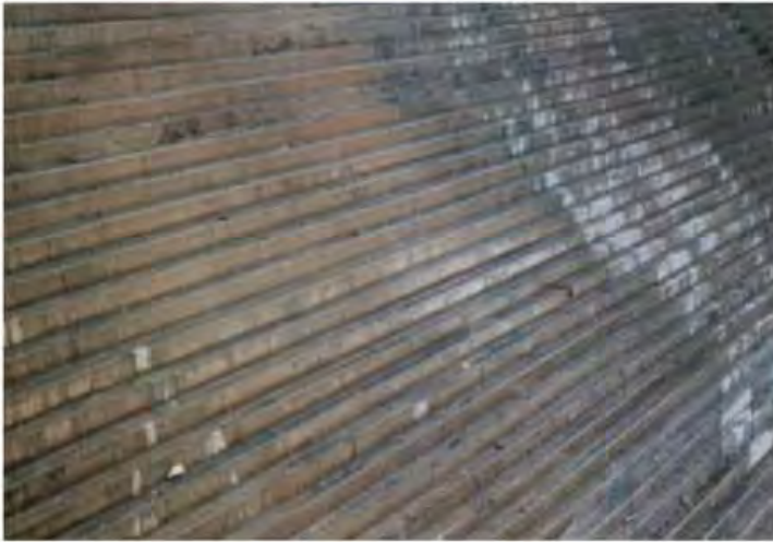
Figure 8.74 CVC poured against the form at a stepped downstream slope - Salto Caxias dam-Brazil.
