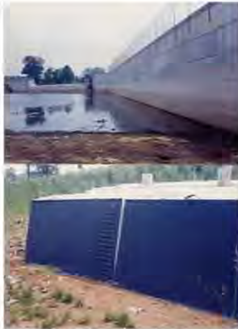
Figure 4.20 Precast concrete panel and the PVC membrane for Winchester Dam,
