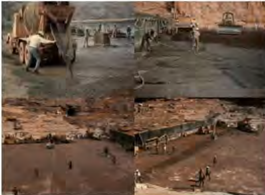
Figure 8.64 Mortar bedding layer being applied on the upstream zone of a construction joint surface, at Capanda dam-Angola.
