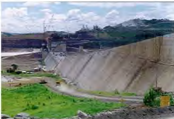
Figure 4.29 Unreinforced stepped CVC concrete at downstream face of Salto Caxias Dam.
