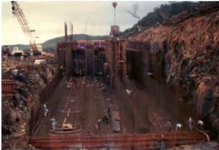
Figure 8.80 Diversion sluiceway built on CVC slipformed at Jordão dam-Brazil.
