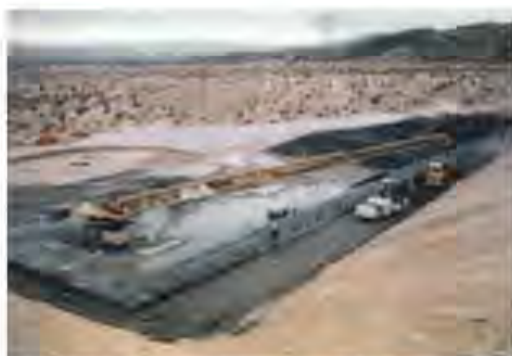
Figure 11.08 RCC used to increase safety during overtopping at Hico Springs Detention Basin. (Courtesy: ROTEC Industries)
