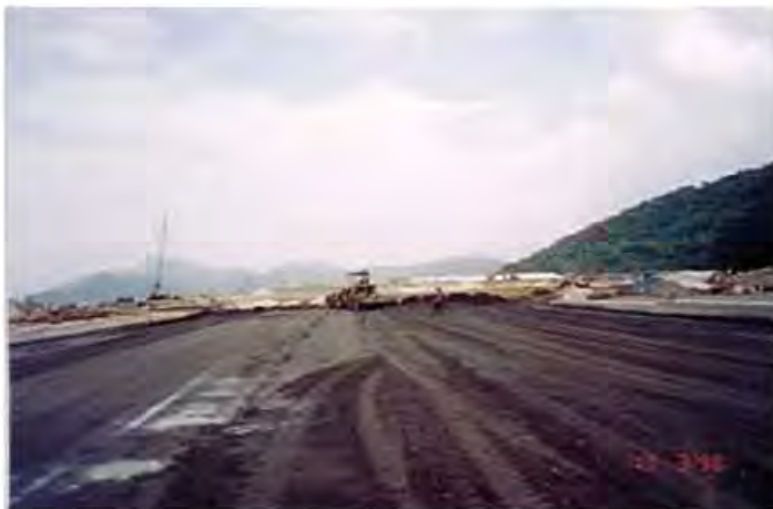
Figure 11.17 Spreading and leveling the RCC (total volume – 84,150m 3 ) for the terminal pavement at Sepetiba bay, Rio de Janeiro State, Brazil. (Courtesy: Carlos Yukio Suzuki-Planservi Engenharia Ltda.)
