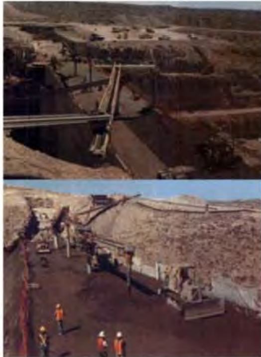
Figure 8.23 Belt conveyor used for RCC transportation and placement at Cuchillo Negro dam (Courtesy: Rotec Industries).
