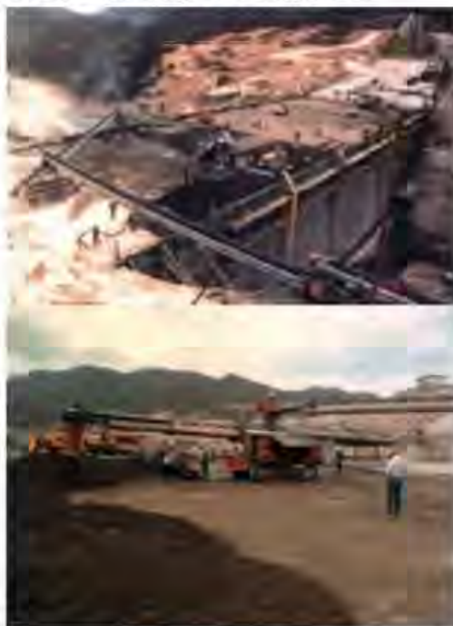
Figure 8.26 Belt conveyor used for RCC transportation and placement at Concepcion dam (Courtesy: Rotec Industries).
