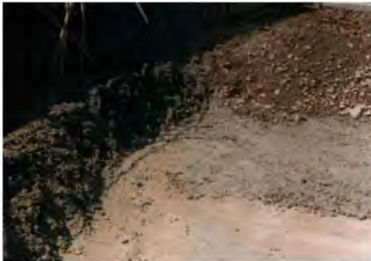
Figure 8.43 CVC mixture being placed in advance with RCC immediately spread against and on top of the sloping unformed face of the CVC, at Capanda Dam-Angola.
