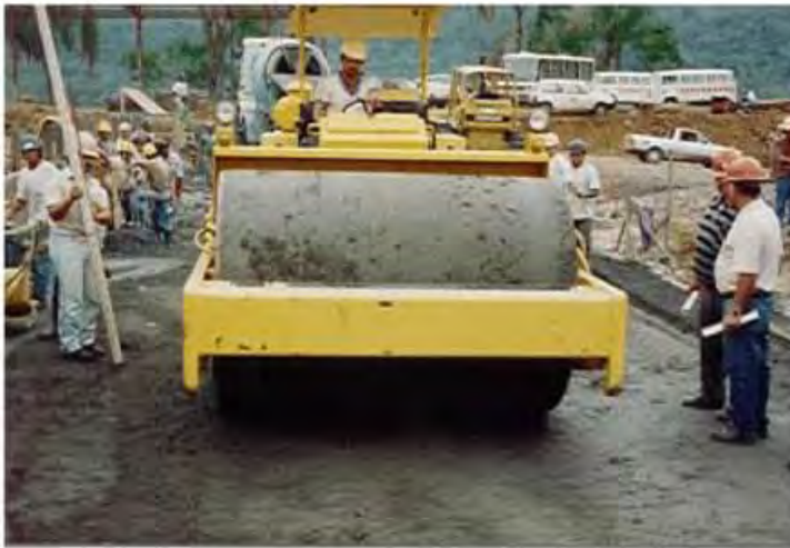
Figure 6.24 Test fill during RCC compaction.
