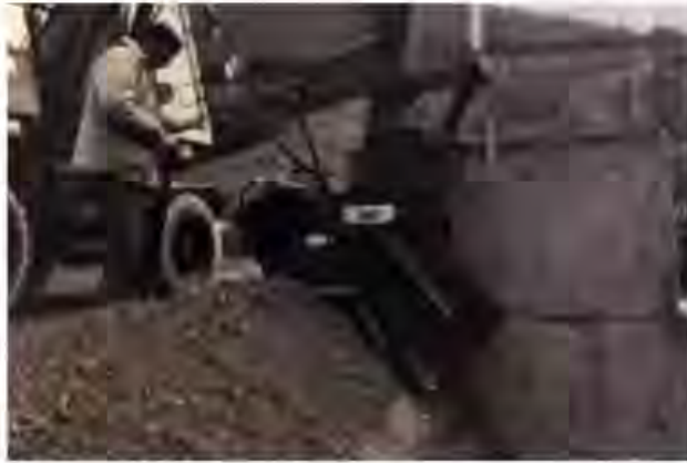
Figure 8.76 RCC in a downstream slope compacted by a special machine.
