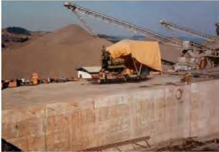
Figure 9.43 Drilling cores from the Test Fill- Jordão Site- Brazil.
