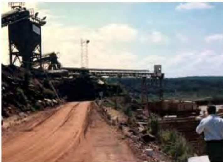
Figure 8.30 Belt conveyor used with a hauling vehicle for RCC transportation and placement at Capanda dam-Angola.
