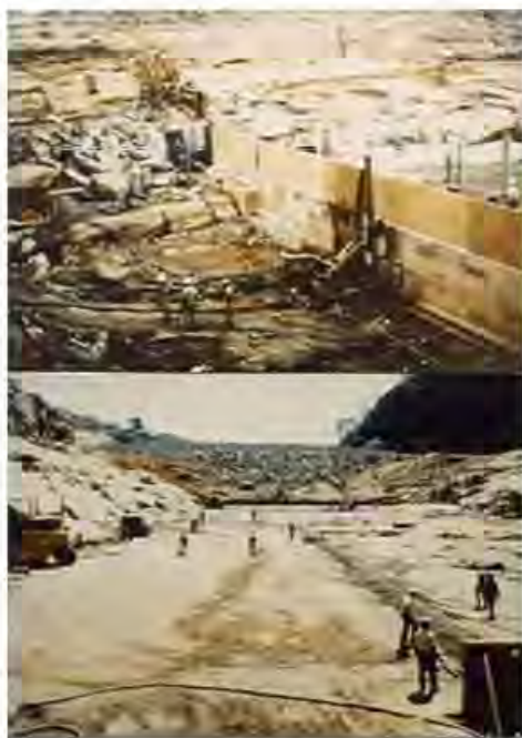
Figure 4.04 Foundation treatment and preparation at Capanda Dam- Angola
