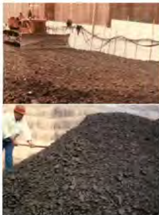
Figure 8.33 Segregation occurred during RCC drop onto the lift surface.
