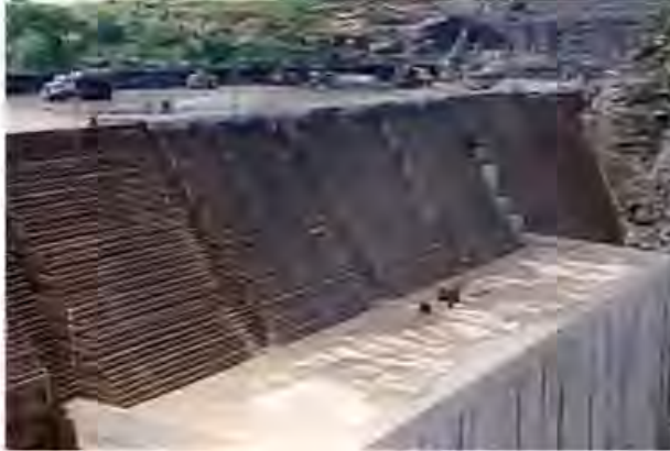
Figure 4.35 Capanda Dam Spillway, during construction. A smoothed CVC concrete face over the RCC mass body provides the surface for the water flow.
