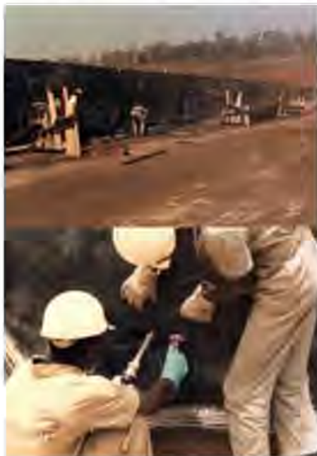
Figure 9.25 Inspection of the PVC Membrane bonding condition at Urugua-i and Capanda Dams.
