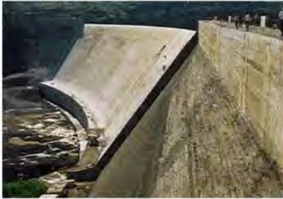
Figure 4.36 Jordão Dam in Brazil – Uncontrolled Spillway. Smoothed CVC concrete surface- Q_{\max} = 7,300 \text{ m}^3/\text{s} .
