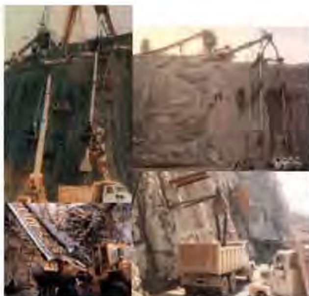
Figure 8.39 Gravity pipe used at Capanda dam-Angola and Jiangya dam-China, for RCC transportation.
