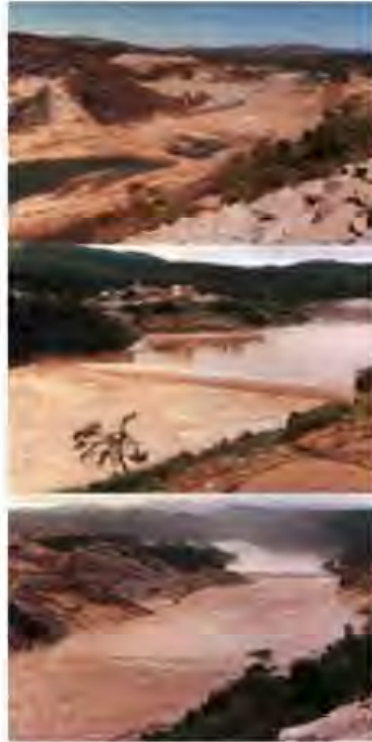
Figure 11.03 Serra da Mesa cofferdam, during one of the overtoppings. (Courtesy: W. Pacelli, FURNAS)
