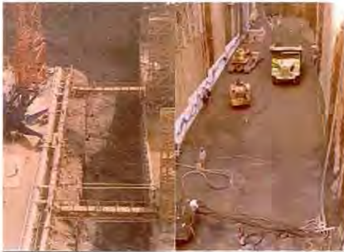
Figure 3.09 RCC used as backfill of an access ramp at Itaipu Project- 1978
