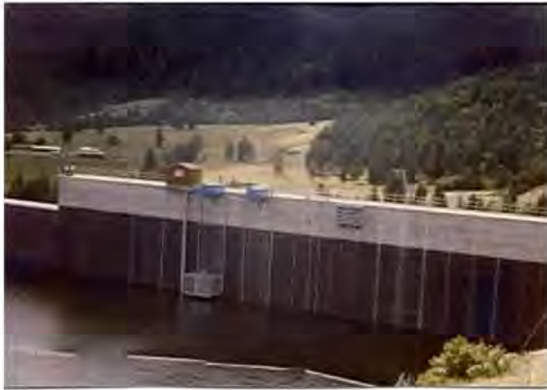
Figure 4.26 Elastomeric upstream membrane at Gallesville Dam (Courtesy: Selmo C. Kuperman).
