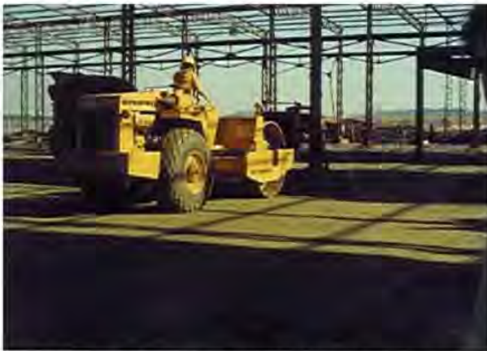
Figure 3.02 RCC used in the floor of a storage building at Itaipu Dam site facilities (1976)[3.22].
