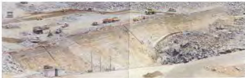
Figure 11.05 Overtopping protection at Xingó Dam during construction, Brazil. (Courtesy: Alberto J. Cavalcanti-CHESF)
