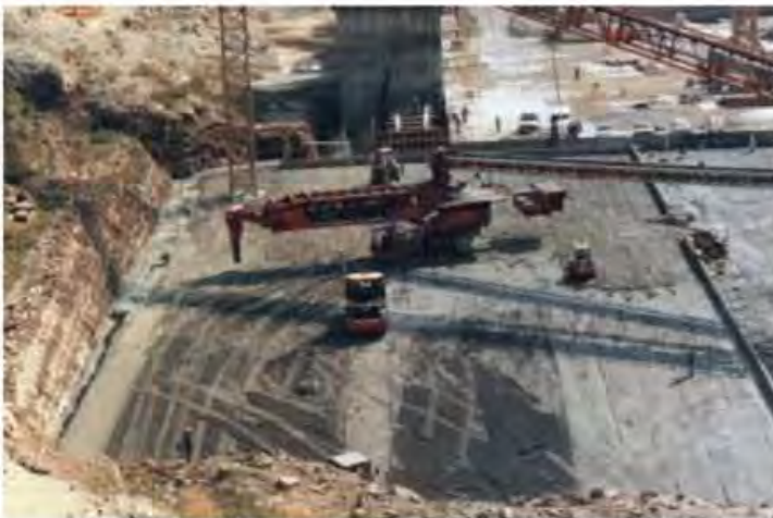
Figure 8.32 Belt conveyor used in conjunction with a “crawler-placer” vehicle for RCC transportation and placement at Rialb dam-Spain.
