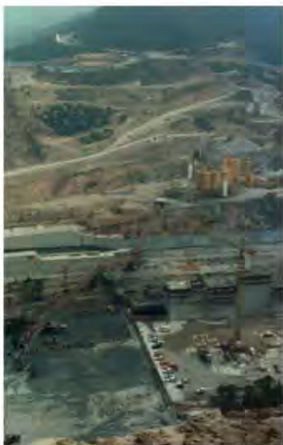
Figure 8.12 RCC batching plant near the center-mass-point, at Rialb dam-Spain.
