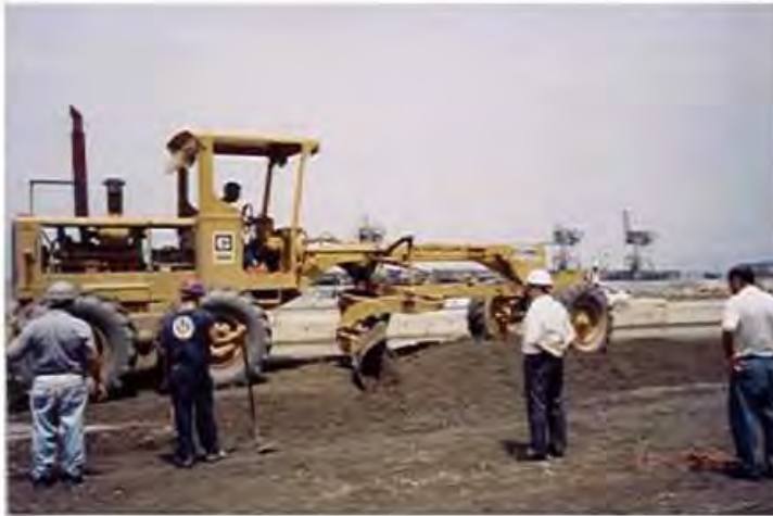
Figure 11.18 Spreading and leveling machine used for RCC pavement at Sepetiba bay, Rio de Janeiro state, Brazil. (Courtesy: Carlos Yukio Suzuki-Planservi Engenharia Ltda)
