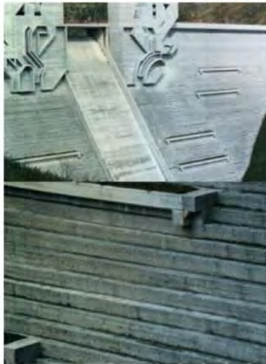
Figure 8.75 CVC casted in a stepped appearance with a pleasing aspect at Arriaran dam-Spain.
