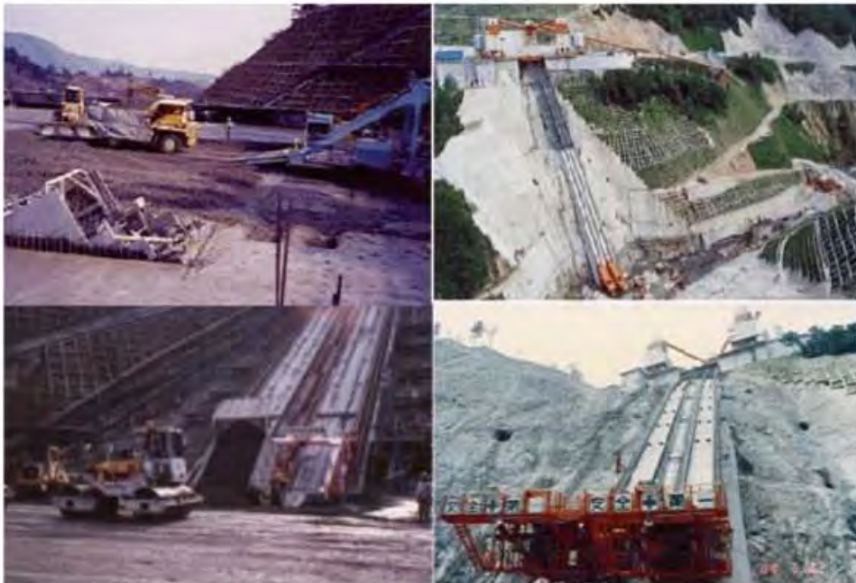
Figure 8.36 System used for handling RCC, at some Japanese dams.
