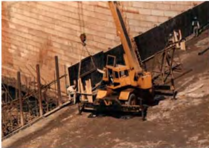
Figure 8.69 Precast element being installed at Urugua-i dam-Argentina.
