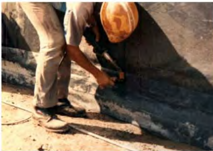
Figure 8.70 PVC membrane being spliced at Urugua-i dam-Argentina.
