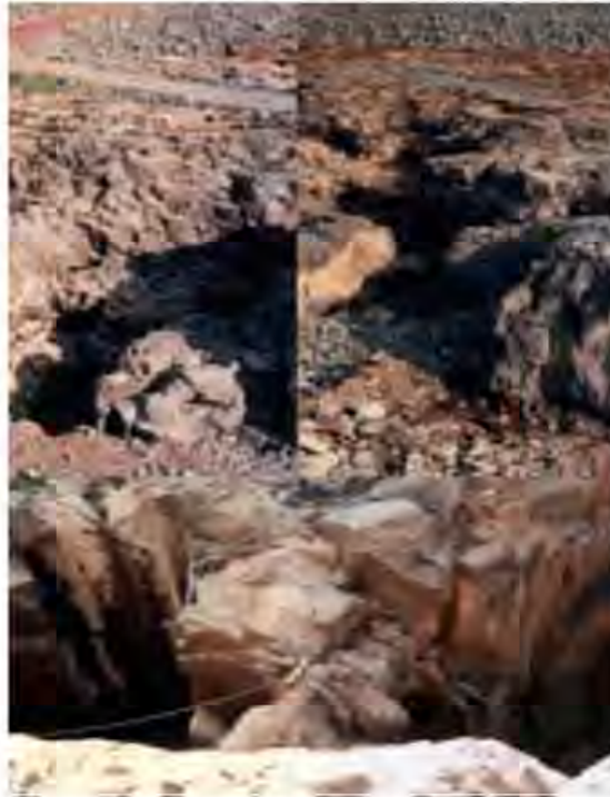
Figure 8.06 If foundation irregularities (holes) have not occurred downstream the sluiceway, but in the area of the RCC dam, a delay in placing the first lifts can be expected.
