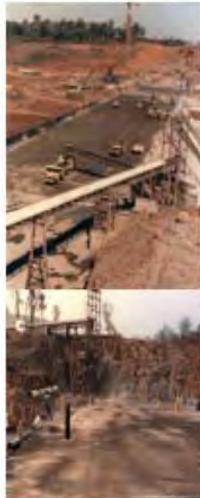
Figure 8.29 Belt conveyor used with a hauling vehicle for RCC transportation and placement at Urugua-i dam-Argentina.
