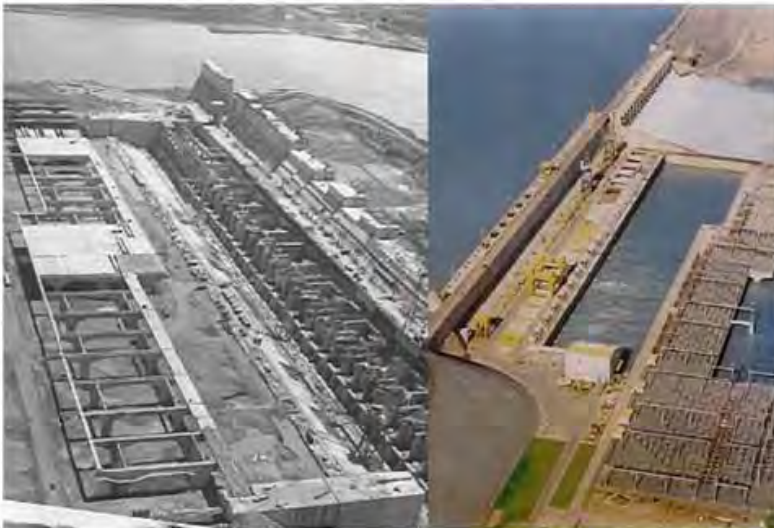
Figure 1.04 Ilha Solteira Hydroelectric Project – 3,620,000m 3 CVC concrete, finished by 1974.
