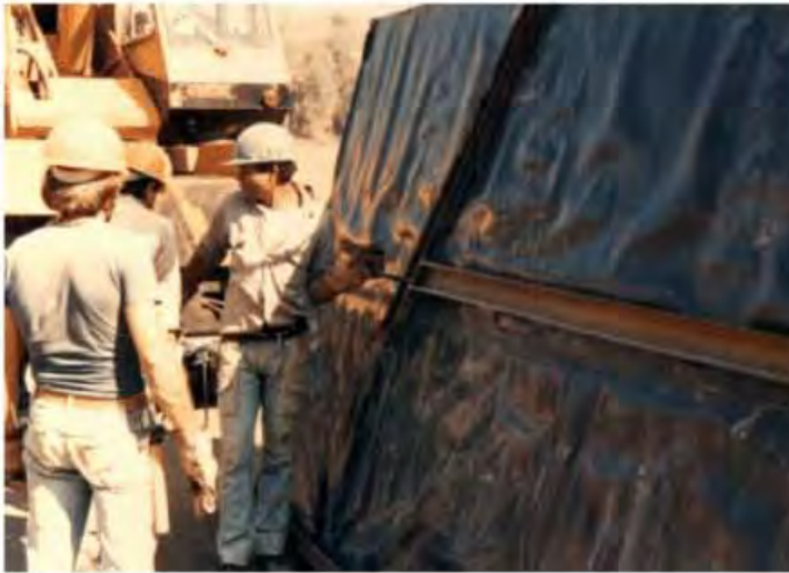
Figure 8.67 Precast element with PVC membrane at Urugua- i dam-Argentina.
