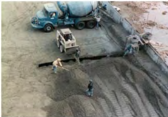
Figure 8.91 Procedure for contraction joint casting at Jordão dam-Brazil.
