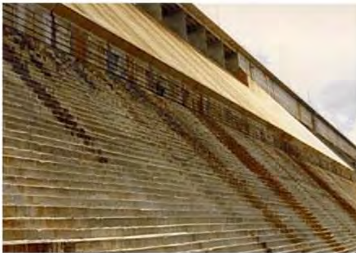
Figure 4.39 Urugua-i Dam in Argentina- uncontrolled spillway. Smoothed CVC concrete surface.
