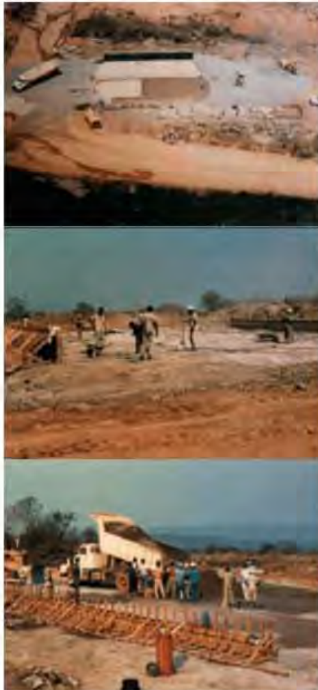
Figure 9.41 RCC placement at the Test Fill- Capanda Site – Angola (1989).
