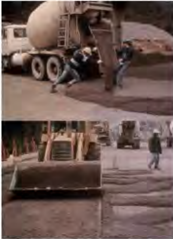
Figure 8.63 Mortar bedding layer being applied on construction joint surface.
