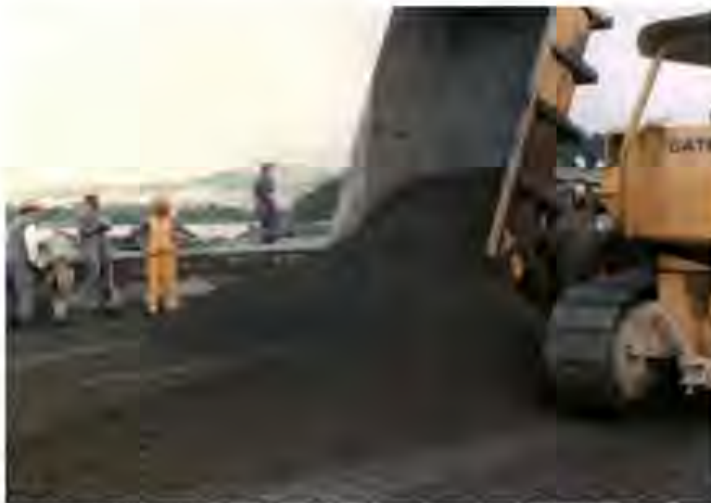
Figure 9.26 Action to reduce the segregation at Salto Caxias dam.
