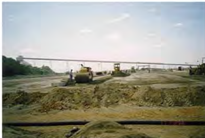
Figure 11.19 Spreading and leveling machine used for RCC pavement at Sepetiba bay, Rio de Janeiro state, Brazil. (Courtesy: Carlos Yukio Suzuki-Planservi Engenharia Ltda)
