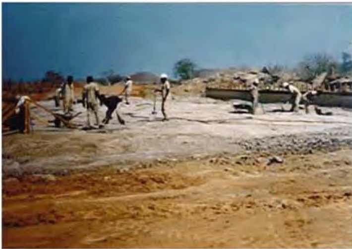
Figure 7.22 Rock surface preparation for RCC test-fill at Capanda job site.
