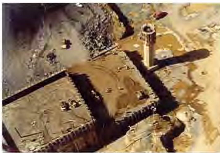
Figure 3.07 RCC placed at the Navigation lock of Tucuruí Dam - Brazil.
