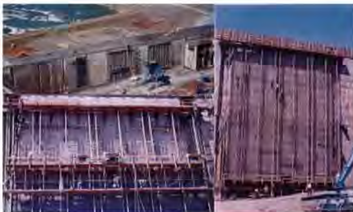
Figure 4.22 Reinforced and jointed concrete face at Salto Caxias Dam, during construction-1996.
