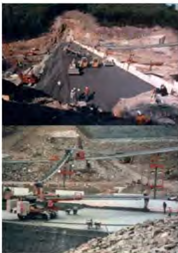
Figure 8.24 Belt conveyor used for RCC transportation and placement at Seigrist dam (Courtesy: Rotec Industries).
