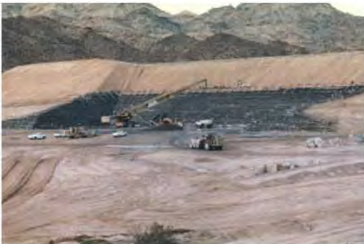
Figure 8.28 Belt conveyor used for RCC transportation and placement at Hicho dam (Courtesy: Rotec Industries).
