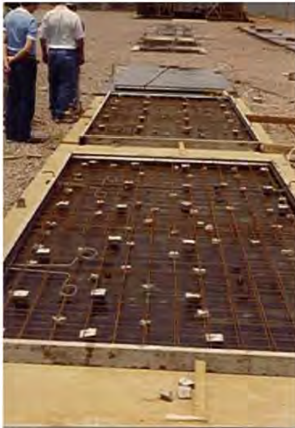
Figure 4.13 PVC membrane inside the panel form at Capanda Dam.
