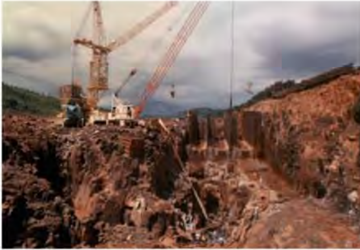
Figure 8.58 Deep holes in the rock foundation at Jordão dam.
