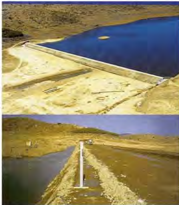
Figure 4.25 Uncompact slopes at Guadalemar Dam in Spain.
