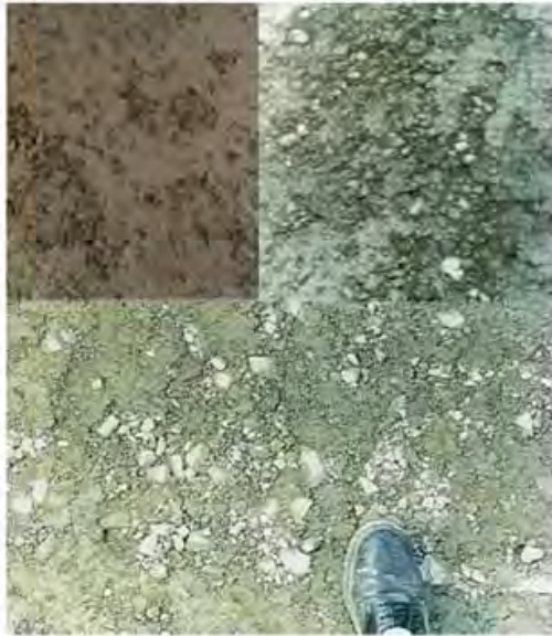
Figure 8.52 Poor texture of RCC surface (opened texture), due to low fines content.
