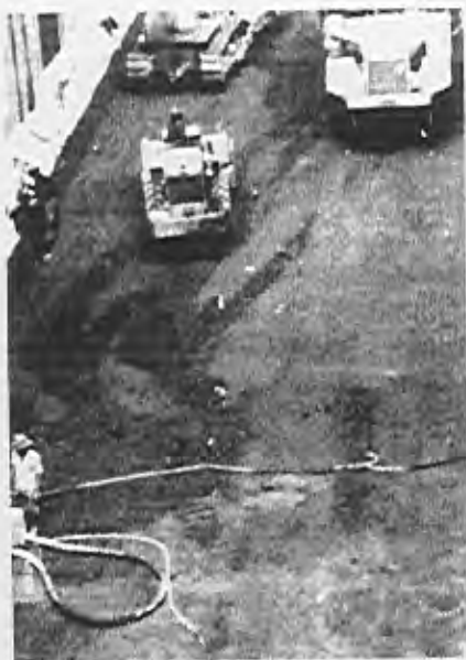
General view of rollercrete placement at the Itaipu project.
