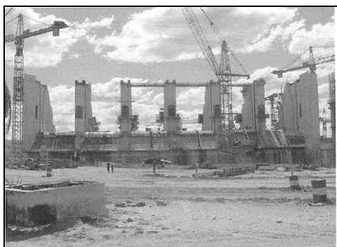
Figure 21 - View of pre-cast beams for Spillway's bridge
