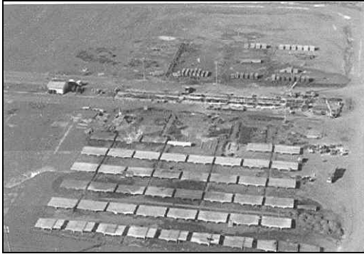
Figure 5 - A pre-cast yard (at Itaipu Project) and the stockage of pieces under final curing
