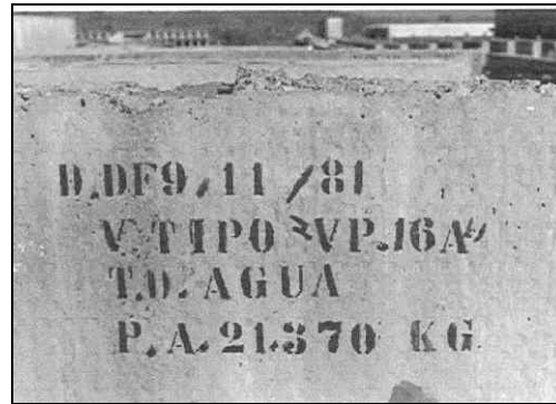
Figure 8 - Pre-cast element identification
