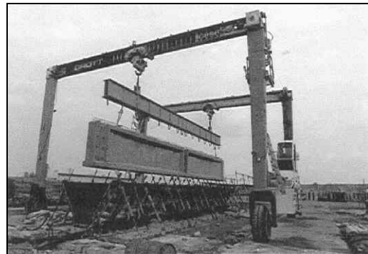
Figure 4 - A long pre-cast element being handled by a special crane
