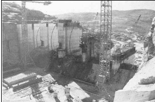
Figure 17 - View of the pre-casts of bridge beam of Spillway - manufacturing area
