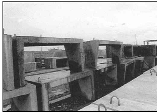
Figure 13 - Pre-cast wall for Instrumentation Hall Building elements Figure 14 - Pre-cast for gallery roof
