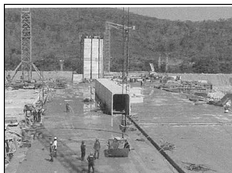
Figure 22 - View of pre-cast galleries for RCC dam
