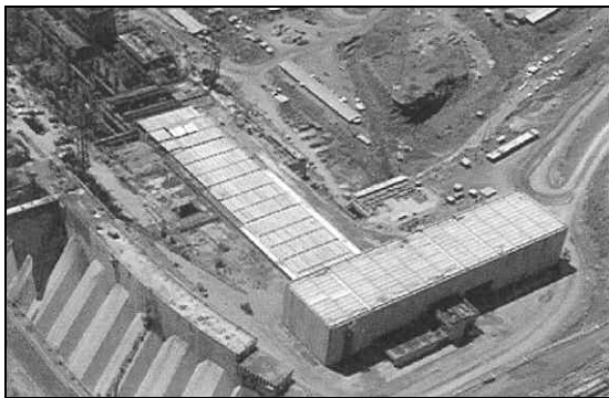
Figure 11 - Assembly Hall Building and Power House Roof constructed with pre-cast elements
