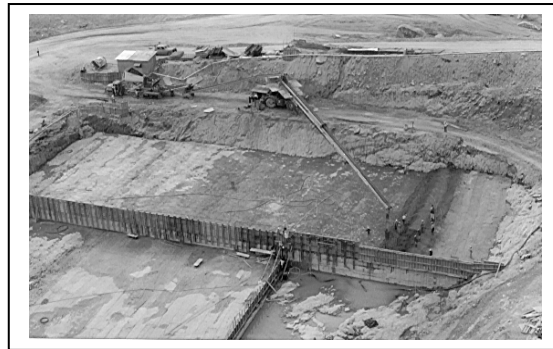
Figure 02-Creter Crane type 200/24-Rotec, handling concrete at Spillway base
