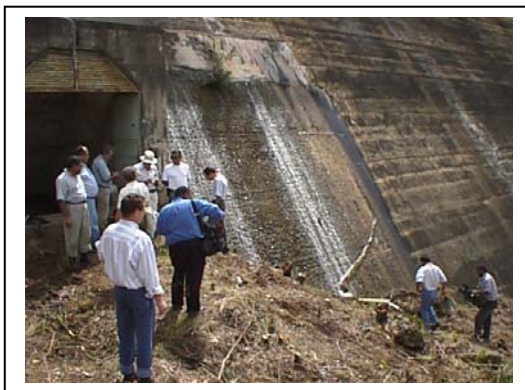
Figure 04- Downstream face of “O” concrete block showing a great leakage
