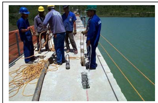
Figure 16- Inspecting the diaphragm panel with TV camera
