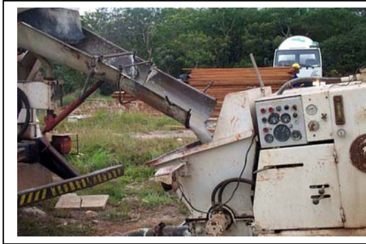
Figure 17- Discharging the mortar from the truck mixer to the placement pump
