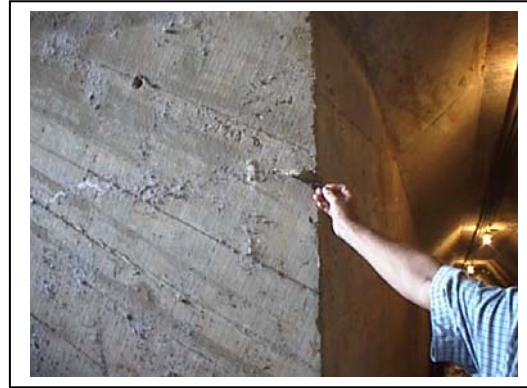
Figure 07- Internal crack in the downstream zone of the gallery flow
