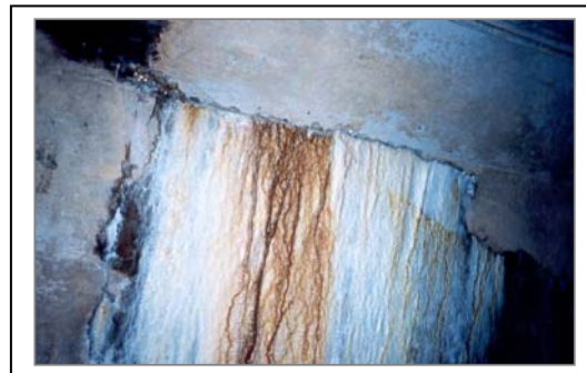
Figure 09- Aggregate reaction at the upstream face of the gallery
