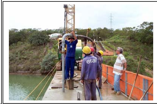
Figure 18- Filling the drilled diaphragm panel with mortar by a “tremie” pipe
