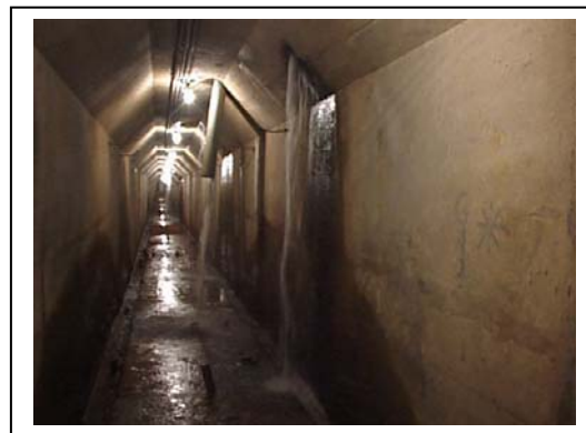
Figure 05- Internal part of the gallery showing the water flow
