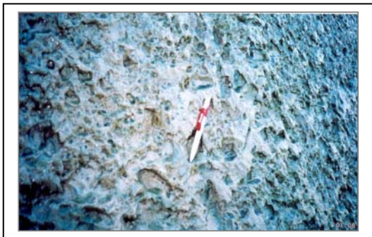
Figure 08- Downstream face of "O" concrete block damaged by aggregate reaction
