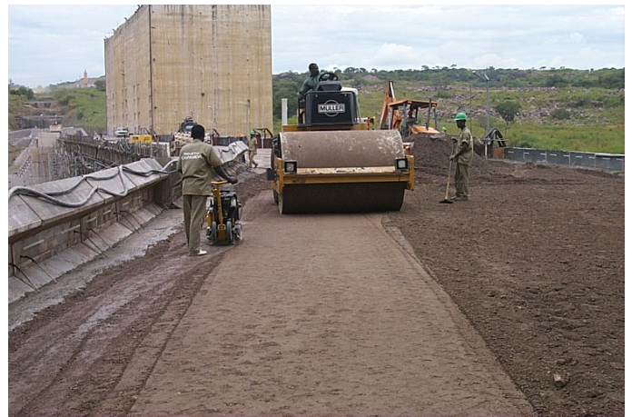
Picture 3 – Compacting of RCC
