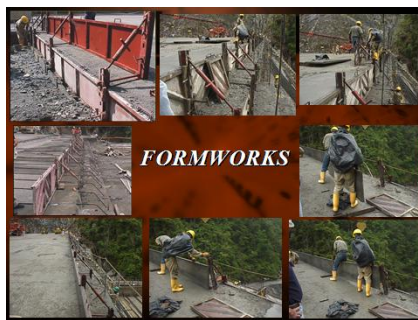
Figures E-43- Metallic Panels that can be used for the Downstream Face
