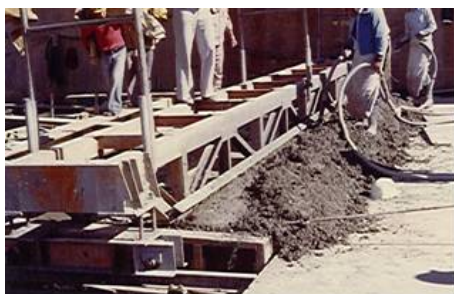
Figures E-44-Straightedge sliding that can be used for the Deflector, Spillway Crest and flatted surfaces
