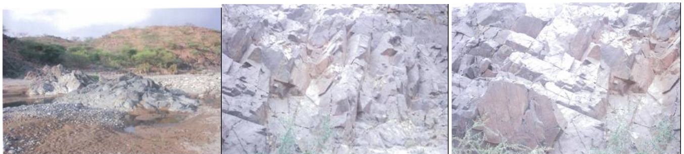
Figure E-30- River Bed Rock and close the River, showing some irregularities (not so smooth surface), that can requires some leveling concrete
