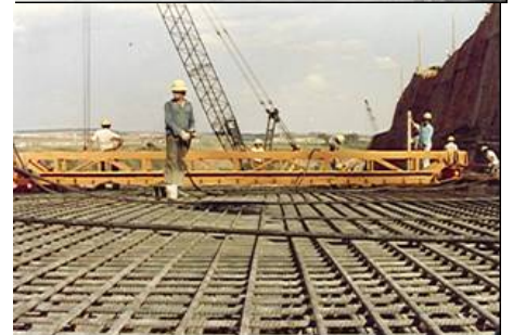
Figures E-44-Straightedge sliding that can be used for the Deflector, Spillway Crest and flatted surfaces
