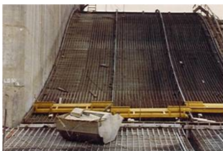
Figures E-43- Metallic Panels that can be used for the Downstream Face
