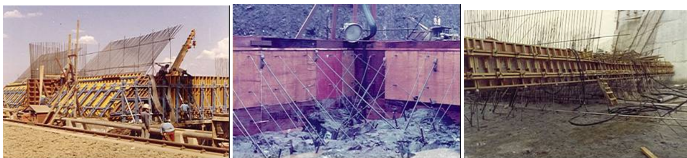
Figure E-40-Wood and Plywood Plane Forms
