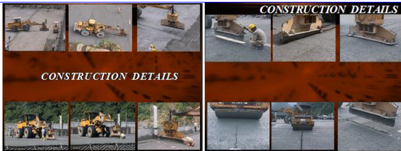
Figure E-39- Casting the Contraction Joint by Joint Inserter machine.
