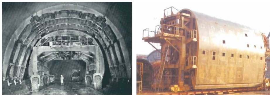
Figure E-46-Tunneling Type Form that can be used for the Diversion Structure
