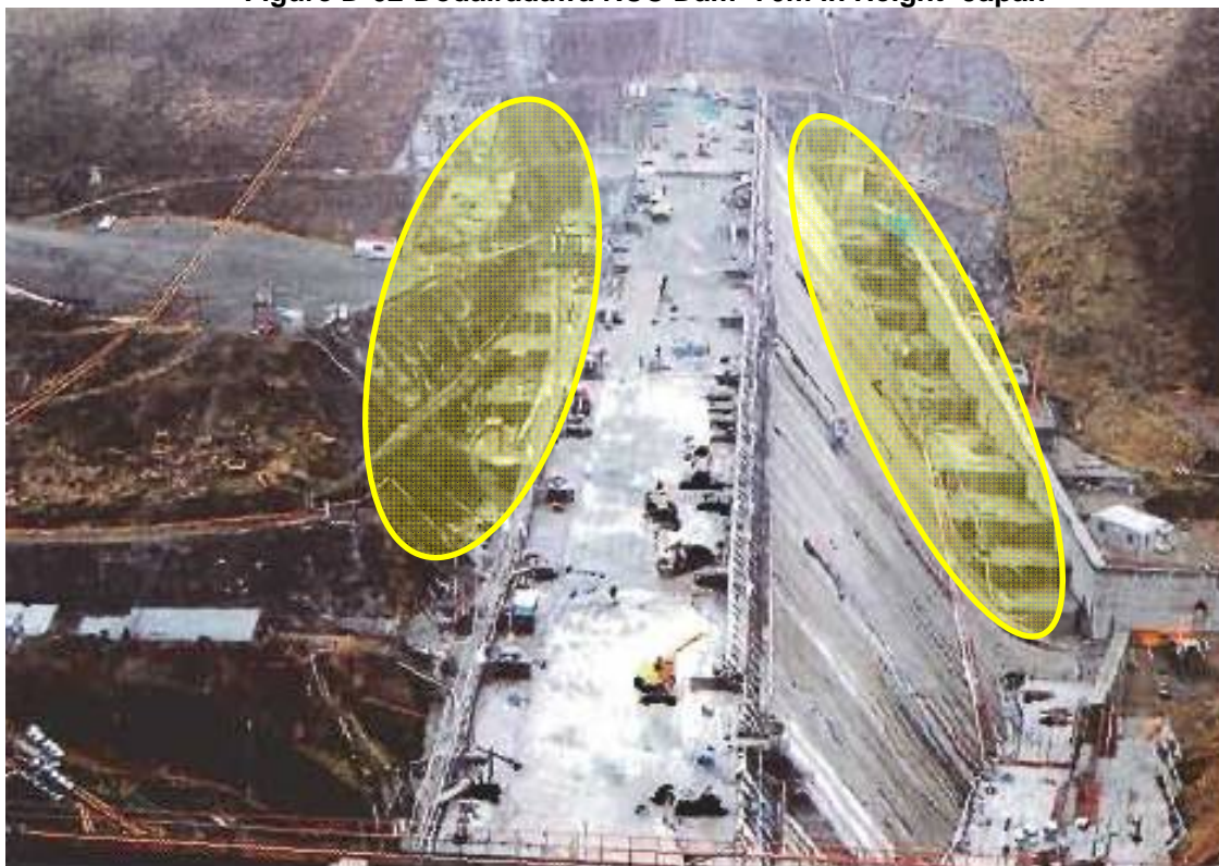
Figure D-03- Enlargement of the dam base at left bank- Dodairagawa RCC Dam – 70m in Height- Japan
