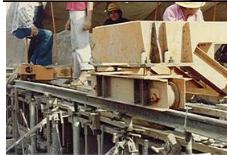
Figures E-44-Straightedge sliding that can be used for the Deflector, Spillway Crest and flatted surfaces
