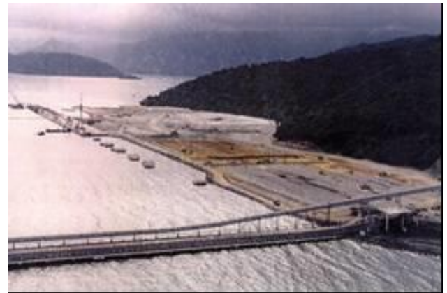
Figure 04- RCC applied in Port Terminal.
