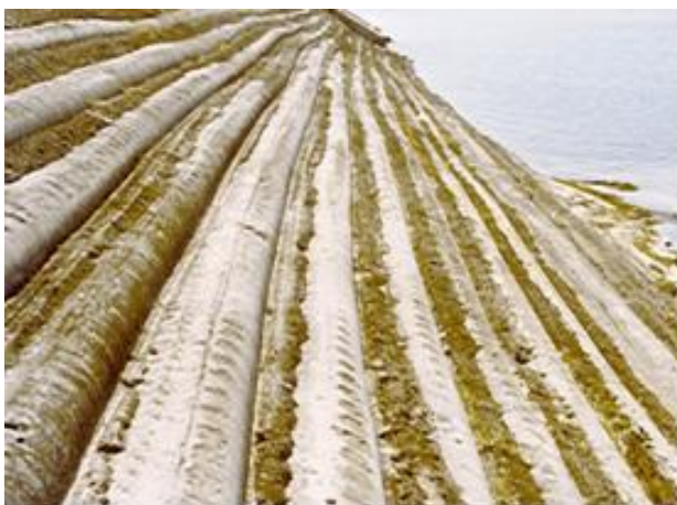
Figure 06- Aspect of the Soil-Cement used as embankment protection in the United States.
