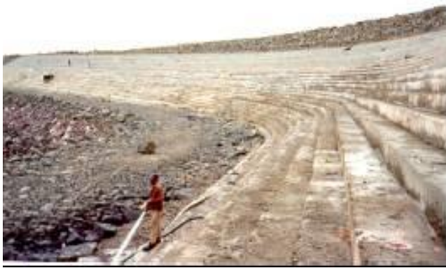
Figure 02- RCC Protection in the Porto Primavera Dam.
