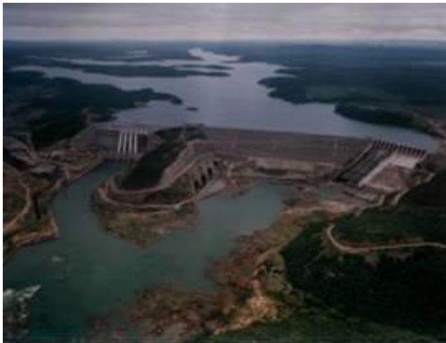
Figure 03- Protection at the region downstream of the of Xingó CFR Dam.
