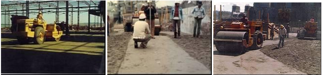
Floor of the Contractor's Warehouse in Itaipu-1976
