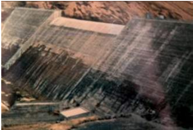
Figure 06 – Willow Creek RCC Dam aspect showing the upstream water level at downstream face
