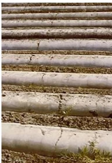
Figure 06 - Appearance of Cracks in the Soil Cement used for the embankment protection of the Martin Dam.
