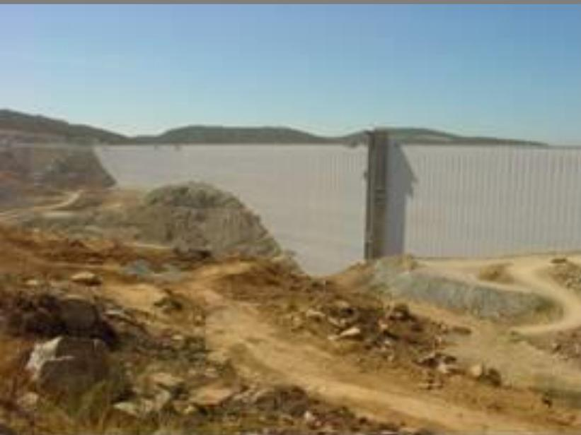
the upstream face. Since the early 1990's, geomembrane liners have and are being used on a higher percentage of RCC dams due to these performance characteristics. Some of the advantages of the geomembrane liner are further described below:
