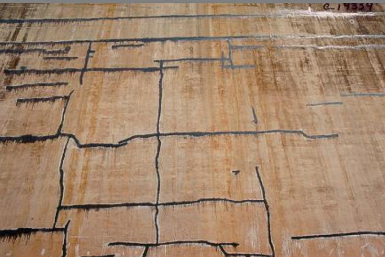
Cracks detected between 0.1 and 0.3 mm were treated with epoxy based sealant (Sikadur 43 enriched with cement), and micro-cracks (thickness < 0.1mm) did not receive previous treatment.
