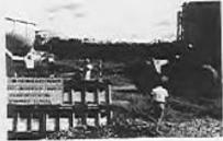
Rollercrete was applied to a permanent structure for the first time in Brazil at the Tucuruí Dam navigational lock.
