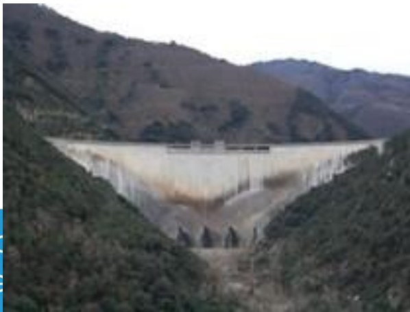
Structural of concrete
